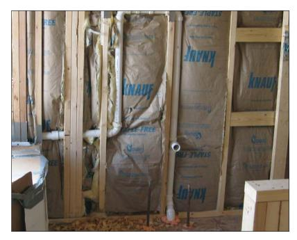
Batt insulation works best when it is fully lofted, not jammed into the tight spaces (left). Compression of the batt reduces the number of air pockets that provide the material's insulation value. It also leaves a hollow between the insulation and the drywall, creating areas where air can circulate. These voids can siphon off energy and may create conditions for condensation and moisture problems.
