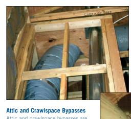
Attic and crawlspace bypasses are penetrations into the living spaces. Pipes, ducts, flues, and electric wires are the most common reason for these penetrations, and the best way to seal them is often (but not always) with ccSPF. Because ccSPF expands and seals, it does an excellent job of filling voids that allow conditioned air to escape. However, ccSPF should *not* be used to seal around high-temperature areas such as combustion appliance flues.
