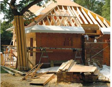
the assembly up, stood it against the tree, and unrolled it around the trunk, securing it with the loose strapping at each end.
