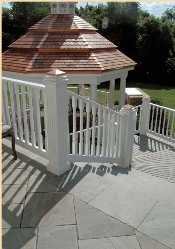
Figure 7. Pavers should be glued to the curbing, and overhang the steps by only an inch to prevent them from being overturned.
