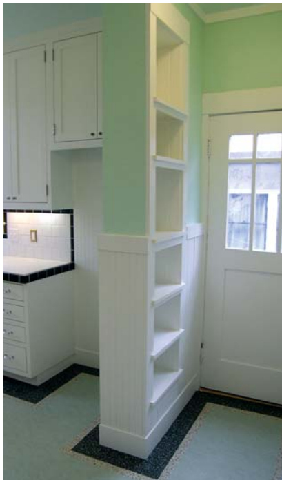
Figure 2. The original water closet's plumbing wall contained pipes for the second-story bath, so it was retained and fattened into a bookcase.
