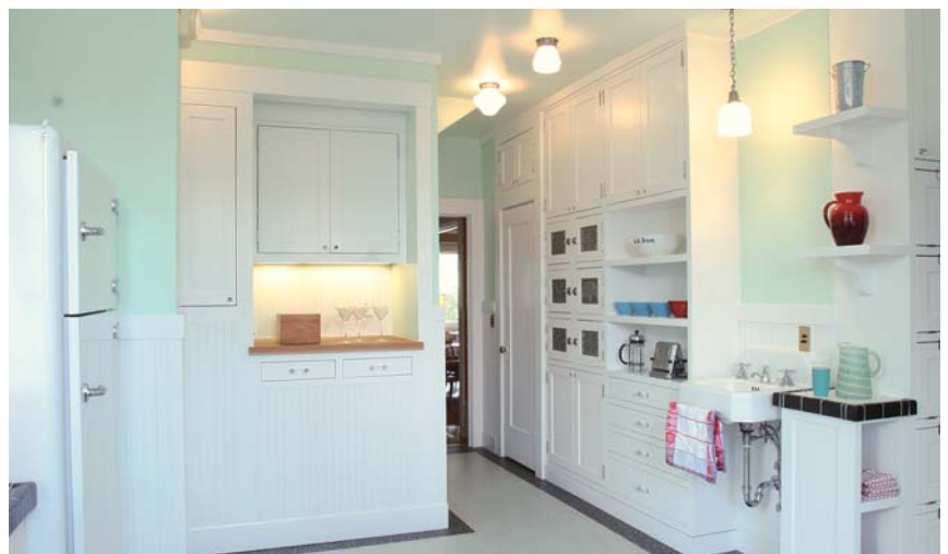
Figure 4. Since a built-in dining room cupboard made 24-inch-deep base cabinets on the kitchen side of the wall impossible (left), the author instead designed shallow apothecary-style cases. Continuous trim ties them to the adjacent closet (below).
