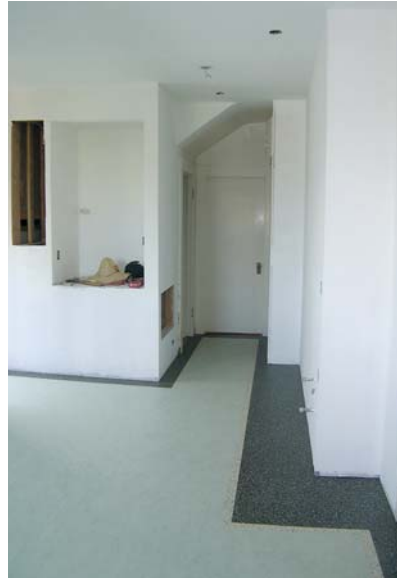
Figure 3. The back stairs (far left) were turned into storage space. The landing became a closet, accessed from the home's main staircase, while the space above the treads now houses a wall cabinet, a niche, and — around the corner — a pair of drawers (left).
