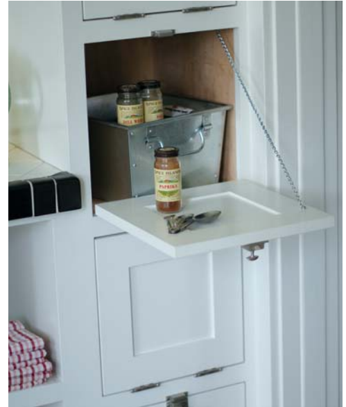
Figure 5. To create a period look, some of the cabinet doors were fitted with inexpensive punched-tin panels (above). Cubbies in the narrow cabinet to the right of the prep sink feature hopper-style doors (right).
