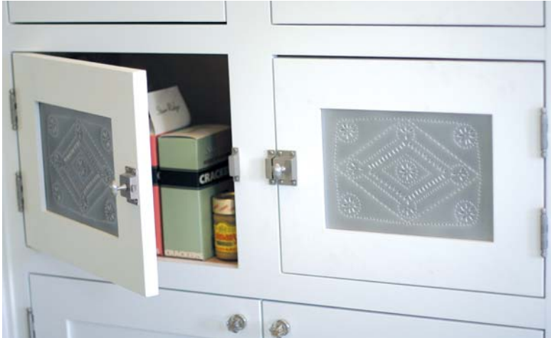
Figure 5. To create a period look, some of the cabinet doors were fitted with inexpensive punched-tin panels (above). Cubbies in the narrow cabinet to the right of the prep sink feature hopper-style doors (right).
