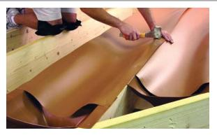
extra outdoor living space, the system protects deck framing from water and thereby helps it to last longer. RainEscape is designed for 12-inch and 16-inch joist spacing and also can be modified for 24-inch on-center spacing. It's guaranteed for 20 years.
