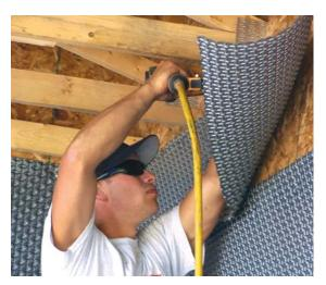
Two for One. Installing rain-screen siding is usually a two-step process: First the housewrap is installed, then the strapping or drainage matrix is applied over it. With *Delta-Dry*, Cosella-Dörken simplifies the process by combining both functions — a water-resistant barrier and a drainage space — into one product. Seams are lapped and then sealed with a companion tape. Available in 39-inch-by-50-foot rolls, Delta-Dry sells for about 70 cents per square foot.
