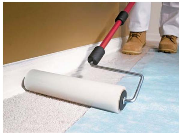
**Easy Roller.** Dispensed from a 9-inch paint roller, *Quick Shield* self-adhering film promises to be a fast and easy way to prep for painting and remodeling projects. At project completion, the film removes without leaving a residue, says the maker. A 100-foot roll sells for \$7.50.
