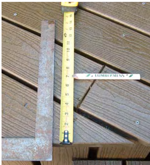
Figure 2. On an existing curved deck, the author locates the posts by measuring in from the deck's edge.
