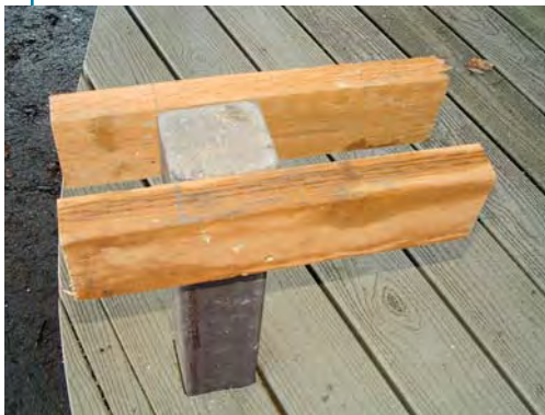
Figure 4. Three screws hold each 2x4 bench support to its post. The inner ends of the 2x4s are run a little long, allowing them to be trimmed exactly after all the seat slats are installed.
