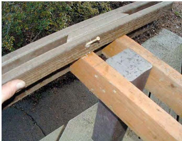
Figure 7. In addition to being screwed to the block behind, each slat is toe-screwed to the 2x4 supports.
