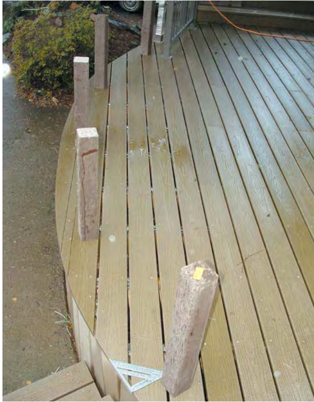
Figure 1. The curved bench will need at least four points of support (three points results in a V-shaped bench). The author has spaced out the posts evenly across the deck to verify position before removing the decking to gain access to the framing.
