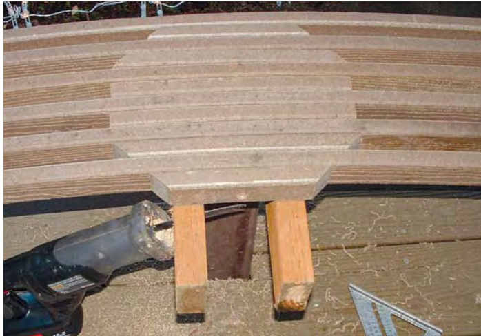
Figure 8. Cutting the spacers at varying angles and lengths results in a circular pattern. The 2x4 supports will be cut off flush with the final block.
