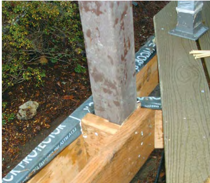
Figure 3. With the decking removed, each support post is nailed in place with blocking on all four sides. If the post lands partially on a joist, notch the post, not the joist.
