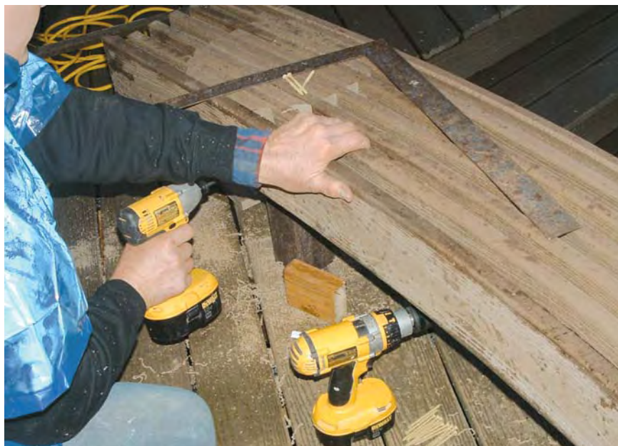
Figure 9. The author screws the inner fascia home.
