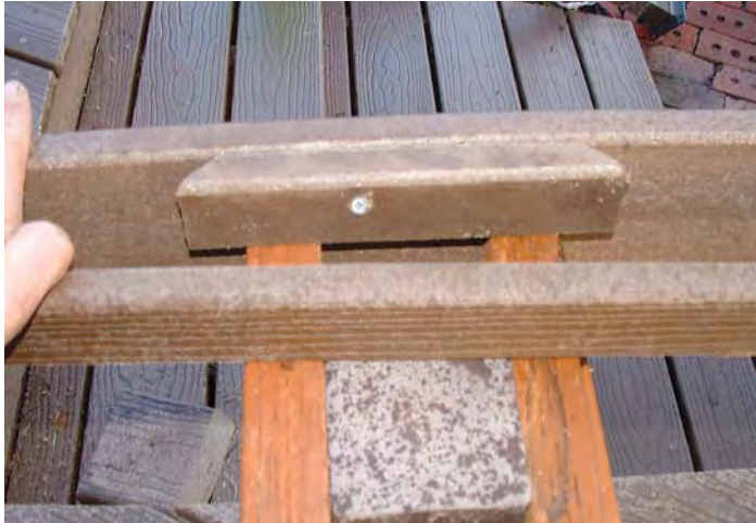
Figure 6. Spacers are screwed to the fascia board above the 2x4 supports, and the slats are bent into place.
