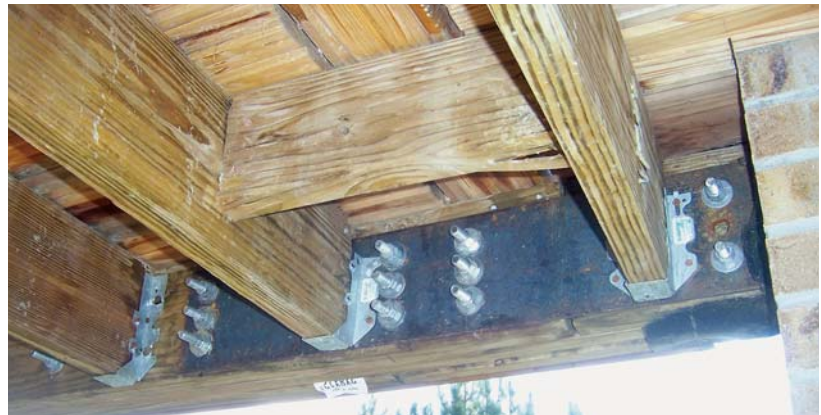
The span called for a three-ply beam, but the carpenter installed only one continuous ply (top). The engineered solution was to add a 1/4-inch flitch plate with twelve 1/2-inch through-bolts (above).
