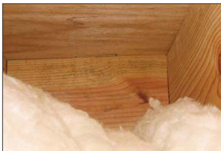
FIGURE 3. Insulation that keeps the subfloor area cool but allows moisture to penetrate exposes the floor to potentially damaging condensation. Over time, the consequences may progress from a small amount of mildew (left) to a major infestation of wood-destroying fungus (right). Before badly damaged wood is protected by more effective insulating material, it should first be cleaned and treated by a capable mold remediation contractor.
