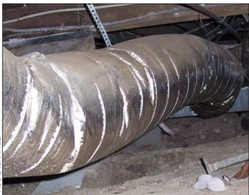
FIGURE 1. Fully enclosed crawlspaces like this one see more severe moisture conditions than open crawlspaces that result when homes are supported by pier and beam systems, reports building science consultant Paul LaGrange. In this example, air conditioning ducts were already dripping condensation in early spring of this year. In general, ducts should be kept out of crawlspaces and placed within the conditioned living space wherever possible.
