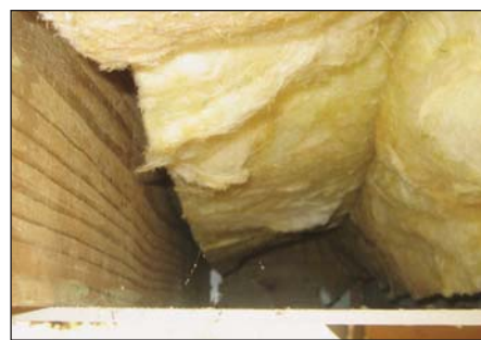
FIGURE 2. Fiberglass insulation installed under elevated floors is typically unprotected and poorly supported. At top, wire mesh has come loose and allowed insulation to fall. In the middle photo, material held up by tacked-on furring strips has become bunched and compressed. The drooping batts at bottom were simply nailed to the subfloor in a few places with cap nails. In all cases, the insulation’s performance is degraded or negated.
