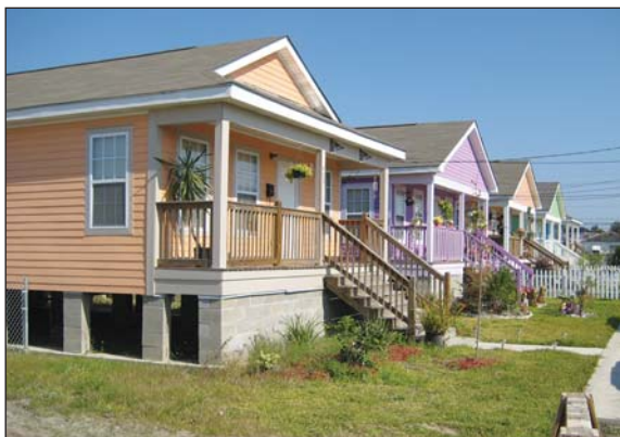
FIGURE 7. Musicians' Village (left), a community of identically built Habitat for Humanity houses in New Orleans' 9th Ward, is the site for a research project into insulation performance in elevated homes. Existing fiberglass insulation, although relatively carefully installed, is still of dubious value in this application. Researchers plan to replace some of the fiberglass with other insulation systems, and monitor the results for a full year.
