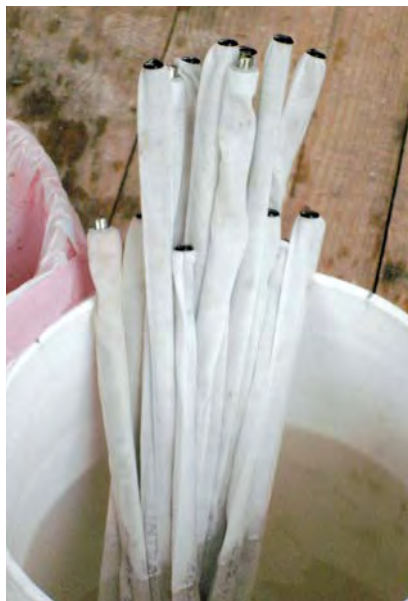
Figure 3. Reinforcing anchors presoak before installation in the masonry. The anchors — hollow, perforated stainless steel tubes in a fabric sock — come in a variety of sizes; the ones shown are 1/2 inch in diameter and 22 inches long.
