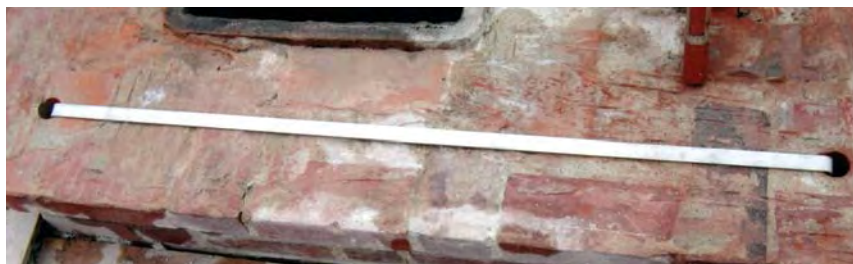
Figure 6. At the top of the completed tear-down level, the author cores down vertically to install stainless-steel reinforcing straps. A wet vacuum prevents the slurry from staining the roof slates below (top left). The straps are site-bent, with 4-inch drop legs, to suit each location (top right). The strap holes are grouted in, while the straps themselves are embedded in the following course of mortar and brick (above).
