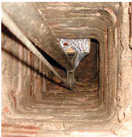
Figure 8. The Ahrens chimney relining process involves drawing a bell-shaped flue-forming device up through a masonry mix that’s added by the bucketful from above. An offset wheel, visible at the end of the 2-inch-pipe, keeps the bell centered in the chase.
