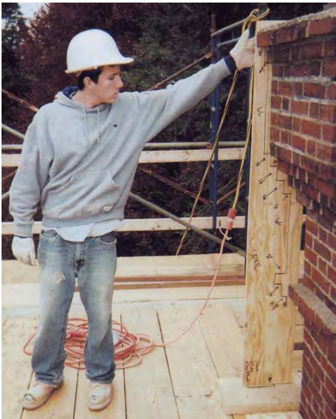
Figure 2. Plywood templates and photography will provide a visual record of the original corbeling when the chimneys are rebuilt.
