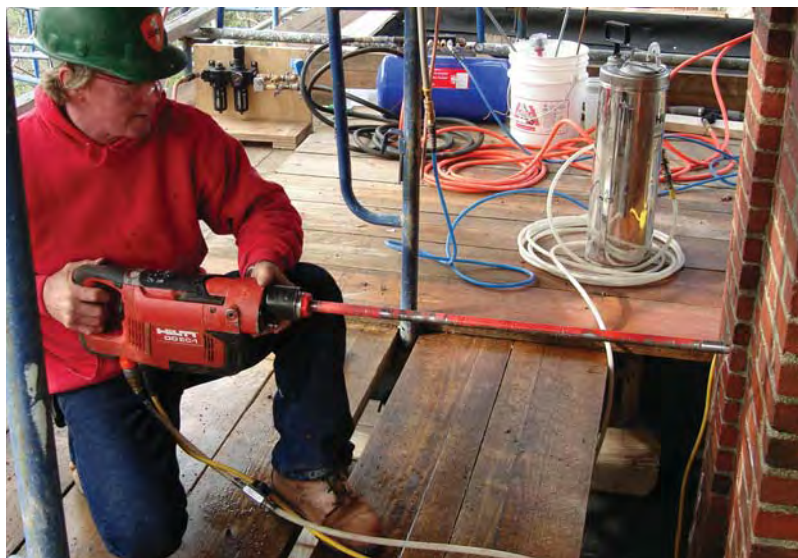
Figure 4. A short 3/4-inch diamond coring bit, guided by a site-made jig, makes the initial hole for the anchors (top). A long-shank coring bit (above) completes the 26-inch-deep holes, providing sufficient depth for the anchors and a finishing masonry core plug.
