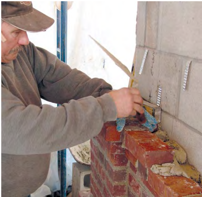
Figure 7. The author uses stainless-steel corrugated wall-ties (about $1 each) and a layup that ensures staggered bonding between bricks. The original work omitted both of these reinforcing precautions.
