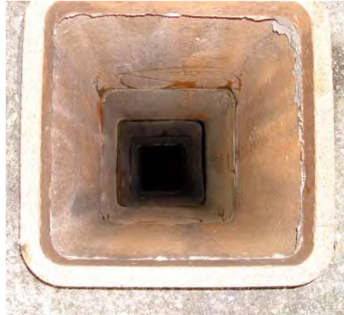
Figure 1. Vertical cracks indicate a chimney in trouble. A combination of water infiltration and unrelieved thermal expansion of the flues caused the failure (far left). The view down the flue shows cracking and water seeping in (left).
