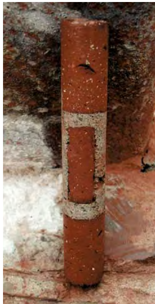
Figure 5. The anchor, fitted with its proprietary mastic injection nozzle, is gently inserted into the cored hole. Grout is pressure-injected until the “grout milk” stops flowing from the site (top). The grout is delivered from a conventional pressure pot at a relatively low psi (above left). The author saved coring plugs to protect and disguise the anchor holes after grouting (above right).
