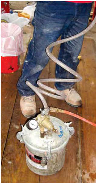
Figure 5. The anchor, fitted with its proprietary mastic injection nozzle, is gently inserted into the cored hole. Grout is pressure-injected until the “grout milk” stops flowing from the site (top). The grout is delivered from a conventional pressure pot at a relatively low psi (above left). The author saved coring plugs to protect and disguise the anchor holes after grouting (above right).
