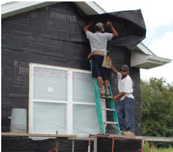
Figure 5. Crew members install a double layer of 60-minute grade D building paper on top of the StuccoWrap (above). The paper laps over a metal weep to allow for drainage at the base of the wall (above right). Galvanized metal lath (right) is then installed over the building paper.
