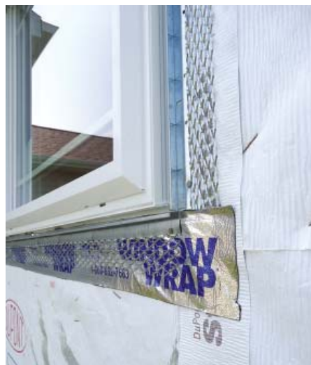
Figure 4. A metal weep screed above the window allows water to drain out from behind the cladding and mortar base coat (left). Metal J-mold is applied underneath the window (above left) and at the jambs (above right); flexible sealant is used to fill the joints between the J-mold and the window.
