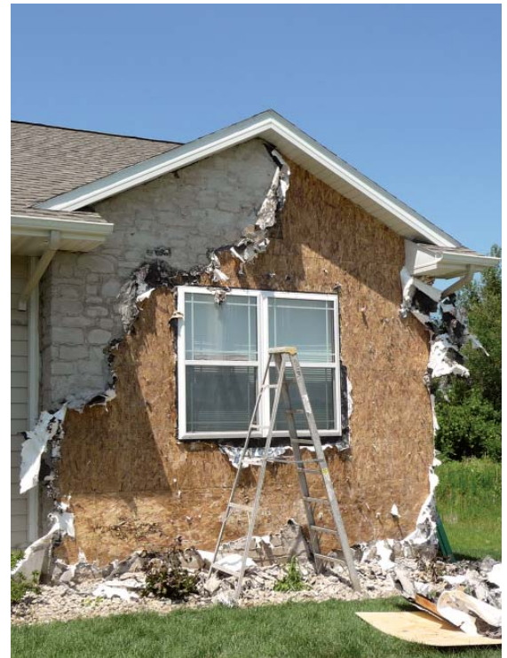
Figure 1. Though it looked sound from the outside, the manufactured-stone veneer on this nine-month-old house was absorbing water and soaking the mortar base coat (left) and the sheathing and framing underneath. The only way to fix the problem was to pull off the stone (right) and install a proper substrate.
