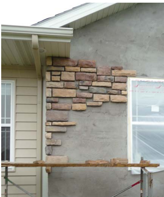
Figure 6. Like stucco, manufactured-stone veneer is applied over a base coat of mortar (left). The cap flashing (above) is sized to match the thickness of the stone veneer, to ensure that water is diverted to the surface.
