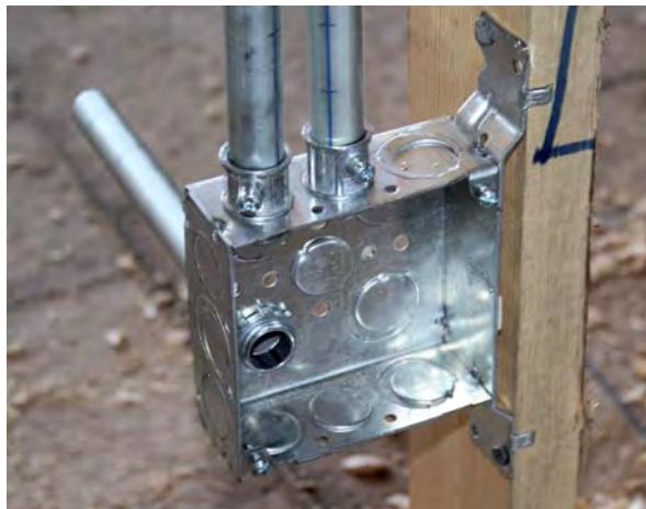
Figure 7. The set screw on a pipe-to-box connector is critical to maintaining a continuous ground. It's securely tightened with a screwdriver or cordless impact driver, and the threaded connection inside is tightened with a knurled lock ring.
