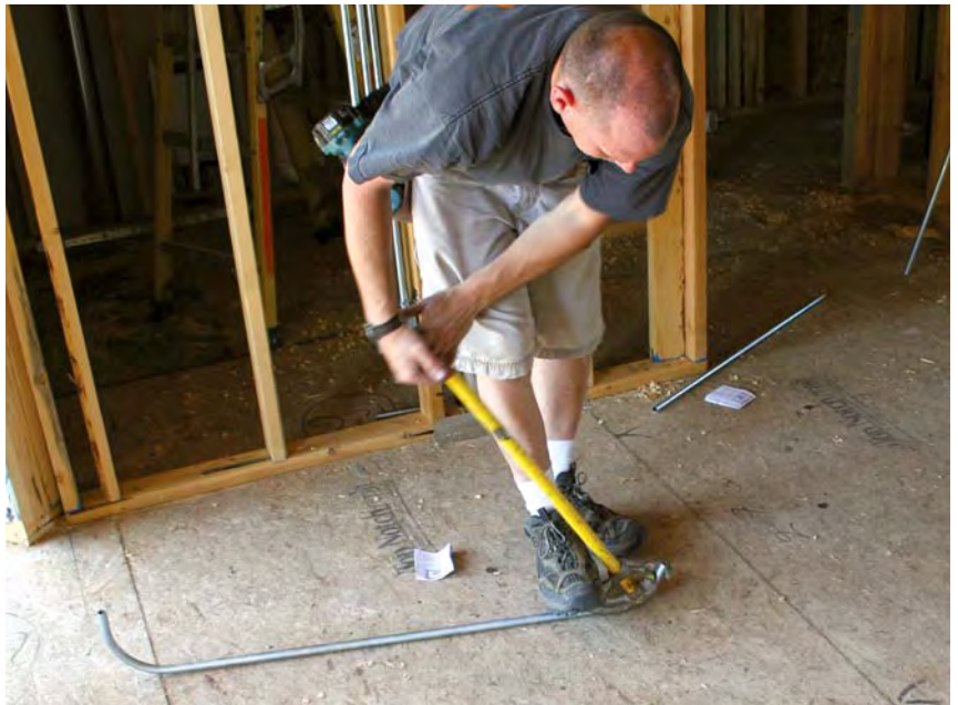
Figure 5. Using the conduit bender as a measuring aid, the electrician marks the location of a bend (top). Then he holds down the pipe with his foot and pulls the bender until the pipe is at the correct angle (above). By hanging the bender from the top of the ladder, he can tweak an angle without getting down (far left). Benders are size specific and come in normal and tight-radius versions (left).
