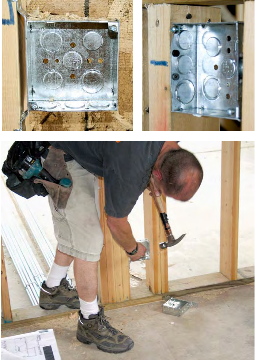
Figure 1. The 4-inch-square steel boxes used most often on residential projects are suitable for switches, outlets, smoke detectors, and light fixtures (top left). Various mounting brackets are available for face and side mounting on wood or steel studs. The boxes also come without brackets, for tight spaces and surface mounting (top right). They're usually attached with drywall screws or roofing nails (above).
