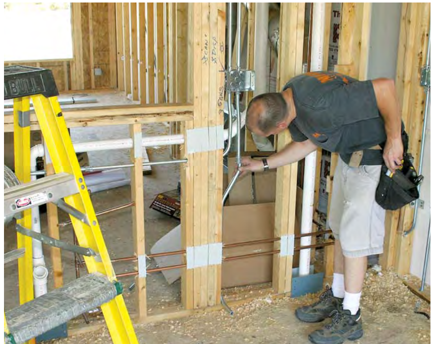
Figure 3. The electrician uses a standard or tight-radius pipe bender to get the pipe to work around obstacles and change directions. Most benders have built-in degree scales, but knowing exactly where and how much to bend the pipe comes from experience.
