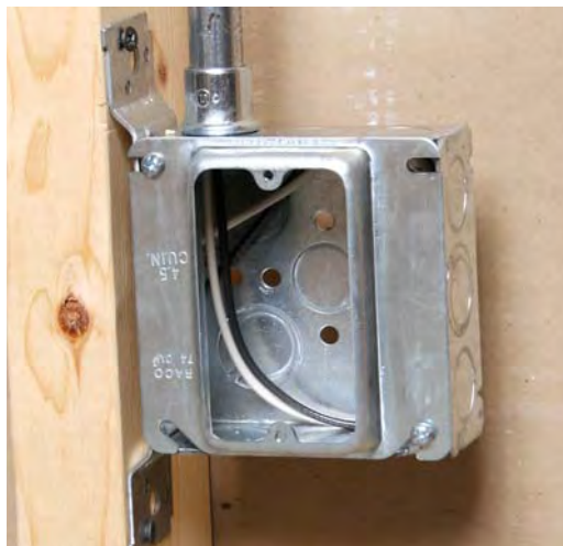
Figure 10. Plaster rings come in one- and two-gang configurations, and in several thicknesses to match a variety of wall finishes. Three- and 4-inch round versions are used for mounting light fixtures and smoke detectors.
