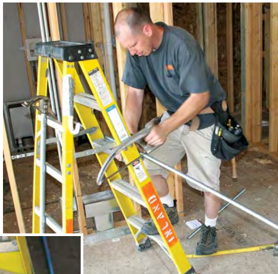
Figure 4. The conduit is generally cut with a hacksaw or cordless recip saw (right). A pair of conduit scraps duct-taped to a rung on the ladder help hold the pipe at a comfortable level (below). Once it's cut, the inside is reamed (below right) so that the burr edge doesn't cut or chafe the insulation when the wire is pulled.
