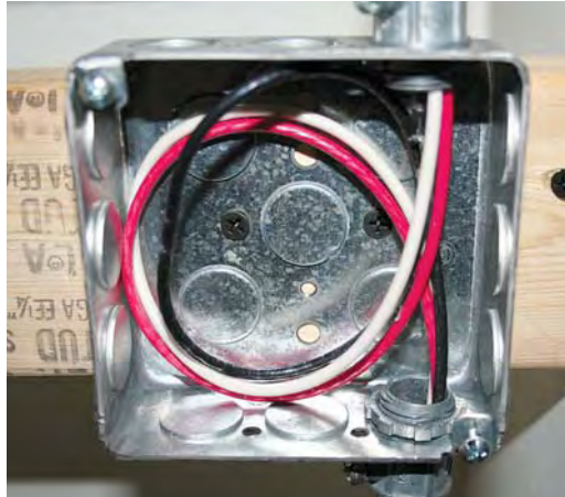
Figure 8. Once the wires are pulled and any necessary connections have been made, the box is ready for a plaster ring. Since one long pull is easier than several shorter ones, the electrician often leaves loops for making the connections and continues the pull.
