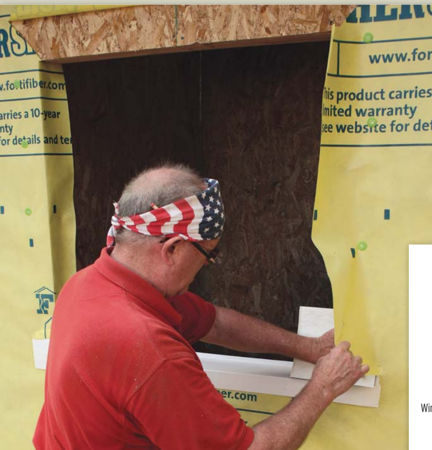
Figure 3. The pan's face flanges tuck under the housewrap (above). As an added measure, peel-and-stick flashing laps over the flanges and end dam. With the housewrap secured by staples and tape, the opening is ready for the window (above right). Note that the pan is installed over sealant, and that the window unit will be pressed into a single bead of sealant at the inside edge of the pan (illustration, right). There should be no sealant directly under the window at the front of the pan — or there should be gaps (weepers) in the sealant bead — so that any water that gets in can drain out.
