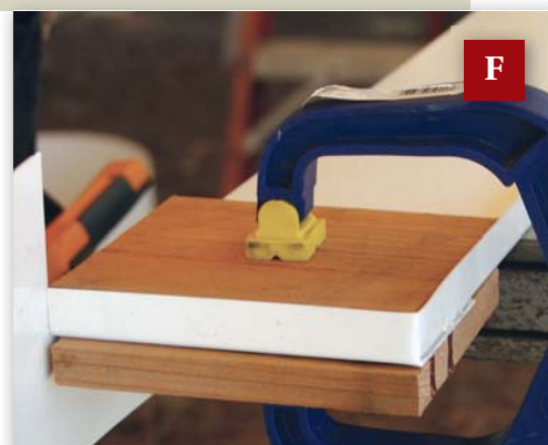
Figure 2. The author slits the bent flashing once down the center and again 4 9 / 16 inches in from the end (A). This allows him to form a face flange (B) and to fold in the end (C) to create an end dam (D). He glues the lap with fast-setting PVC cement (E), clamping the joint until the glue has cured (F).
