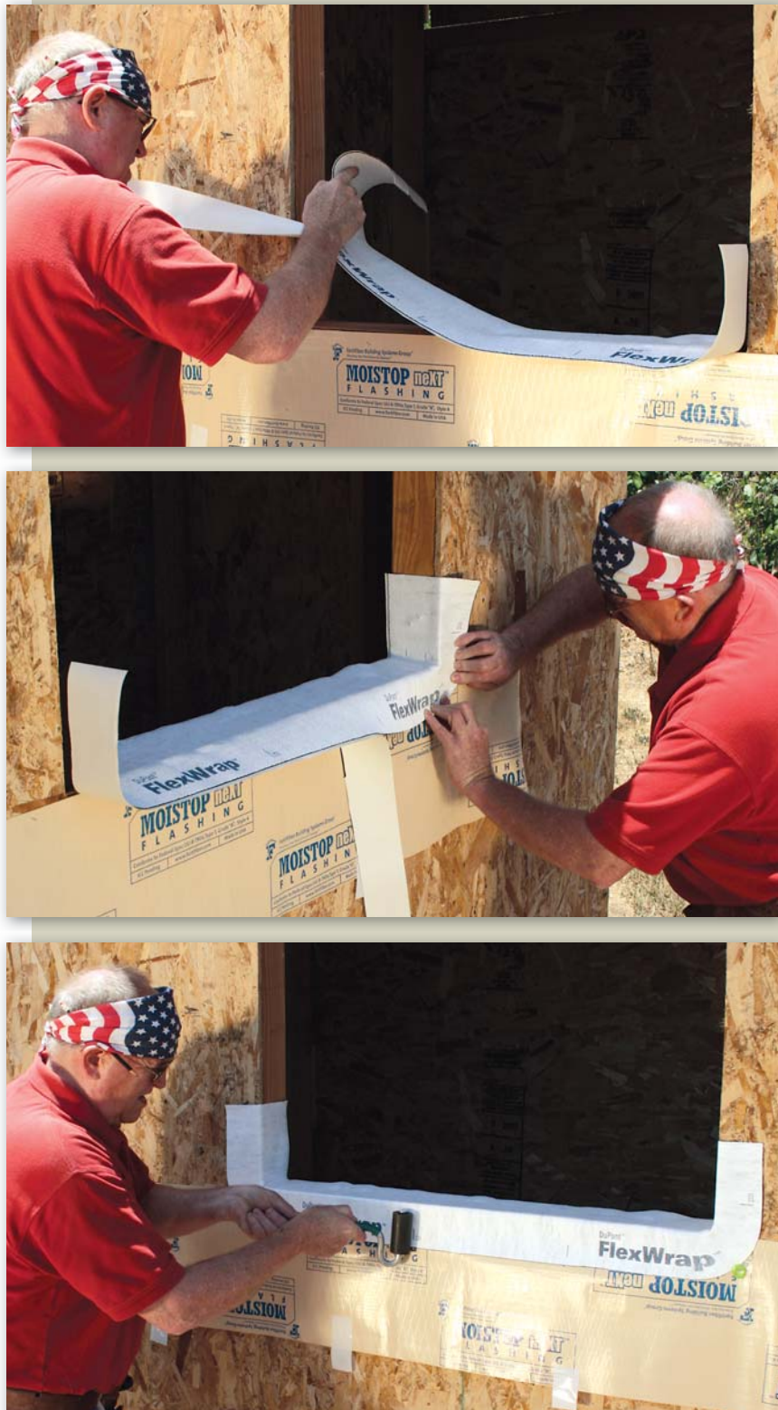
Figure 4. Because this house will be finished in stucco, the sill pan goes in before the building paper, which will tuck under the apron flashing below the window opening. The author installs the pan by adhering flexible flashing to a beveled strip on top of the sill (top), then stretching it around the corners of the opening (center). After stapling the pan to the face of the sheathing, he rolls the entire surface to ensure a good bond (above).
