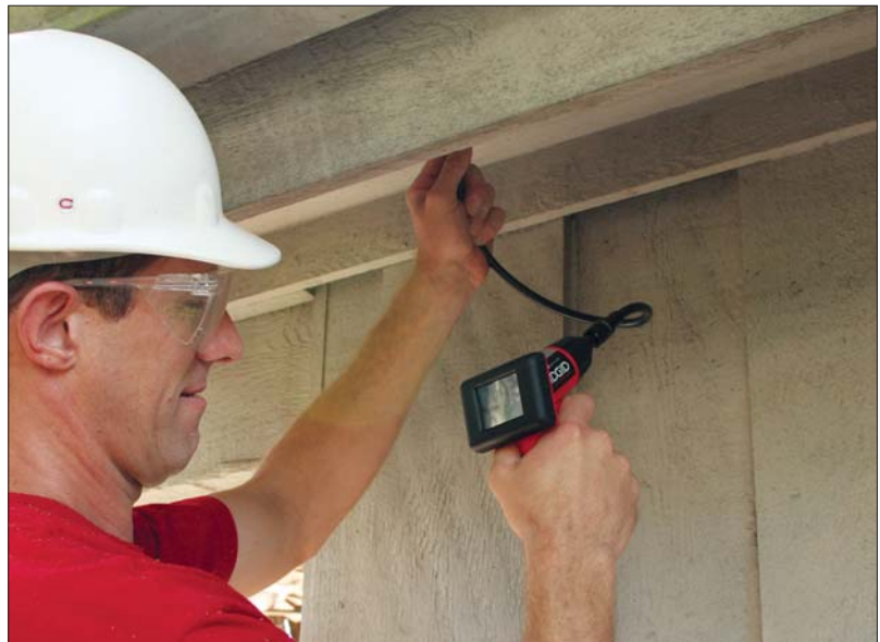
FIGURE 4. Contractors can inspect the roof connections through a small hole in the soffit, using an inexpensive camera probe. A 1.5- or 2-inch hole (top) is sufficient for inserting the probe, which displays a view on a small screen (middle). Aluminum louvers or plastic plugs can unobtrusively cover up the hole. If the connection is sufficient, retrofit won't be necessary. The probe shown here is the Ridgid SeeSnake Micro.
