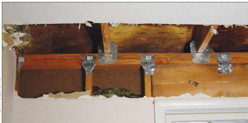
FIGURE 3. Here, steel connectors have been added at stud-to-plate joints as well as truss-to-plate joints, greatly increasing the uplift resistance at these points. However, Florida code requires only the roof connection upgrade, not the wall reinforcement. The clips used here are Simpson H1 clips, which can handle over 1,000 pounds of uplift.
