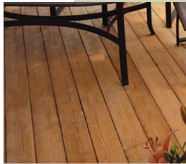
Figure 2. The second generation of preservatives, MCQ and MCA, are less corrosive than ACQ and CA and leave the wood looking closer to its natural color.
