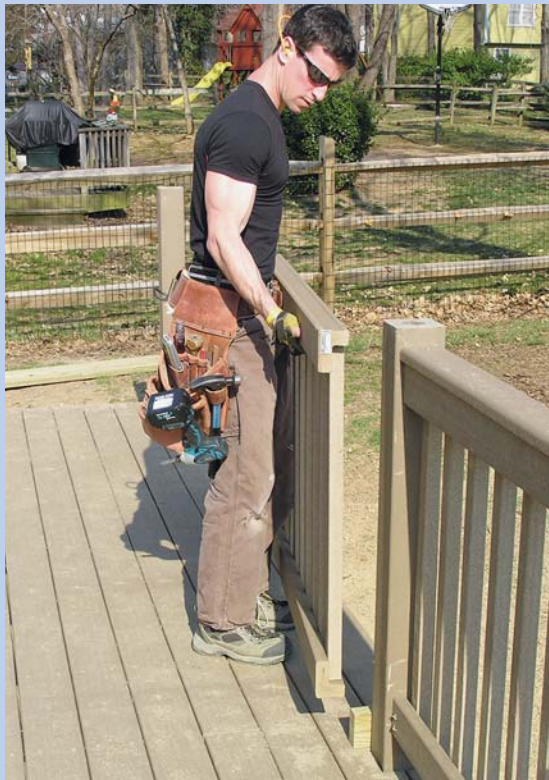
Figure 12. With a 3½-inch toe space, you can rest the rail on 2x4 blocks for support while fastening it.
