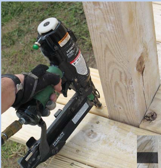
Figure 7. Using 4x6 wood posts eliminates the need to notch the ends of boards. Lay out the final location of the posts as you run the decking so that the boards and the posts are aligned. Construction adhesive and finish nails hold the outboard piece of decking in place.
