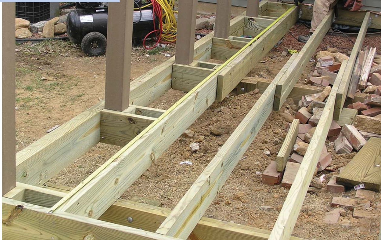
Figure 1. Housings assembled from joist stock and tied into the framing provide stout anchors for guardrail posts. Make the post opening a little big and cut the blocking a little short so it doesn't force the outer joist out of line.
