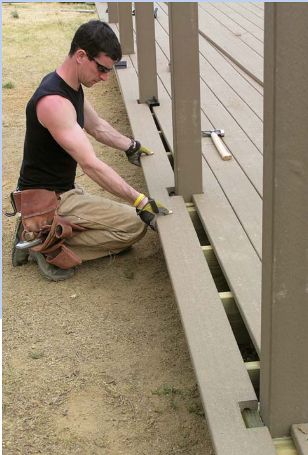
Figure 8. The last board always requires notching. Drill the corners of the holes first, then use a jigsaw to cut out the notches.
