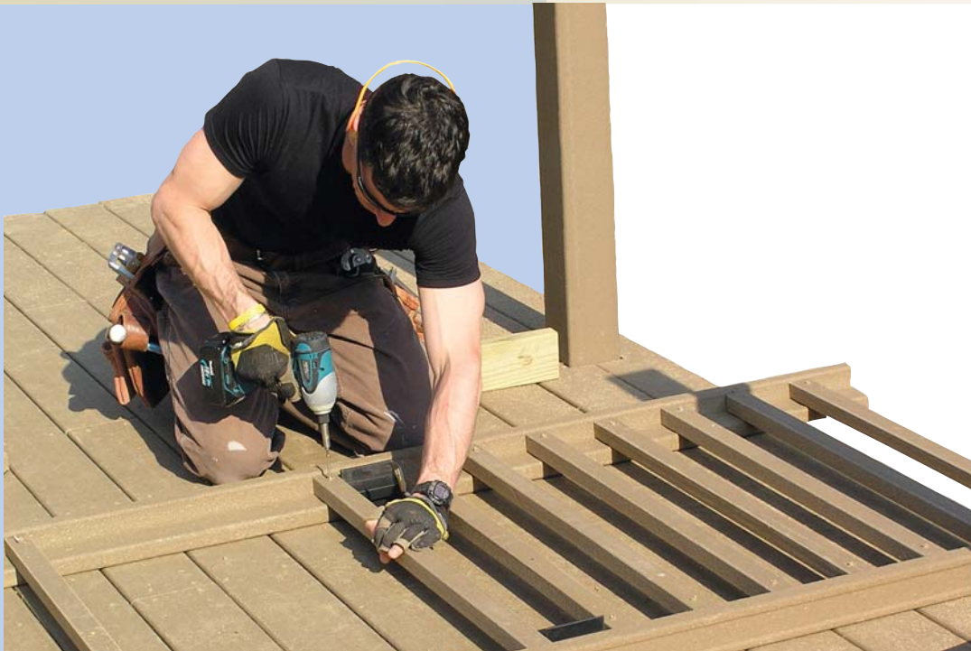
Figure 10. MoistureShield's rails are L-shaped and the balusters are face-screwed in place.
