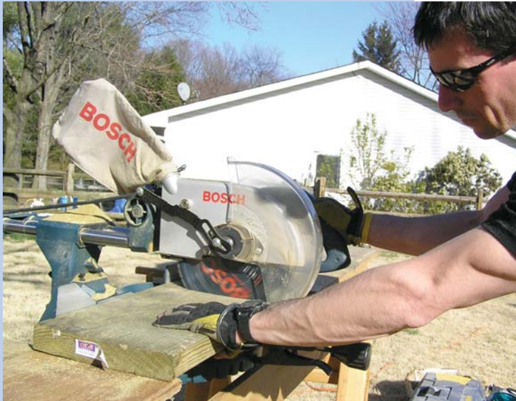
Figure 2. It takes a little extra time in the morning to set up a miter saw, but it pays dividends of fast and accurate cuts all day long.
