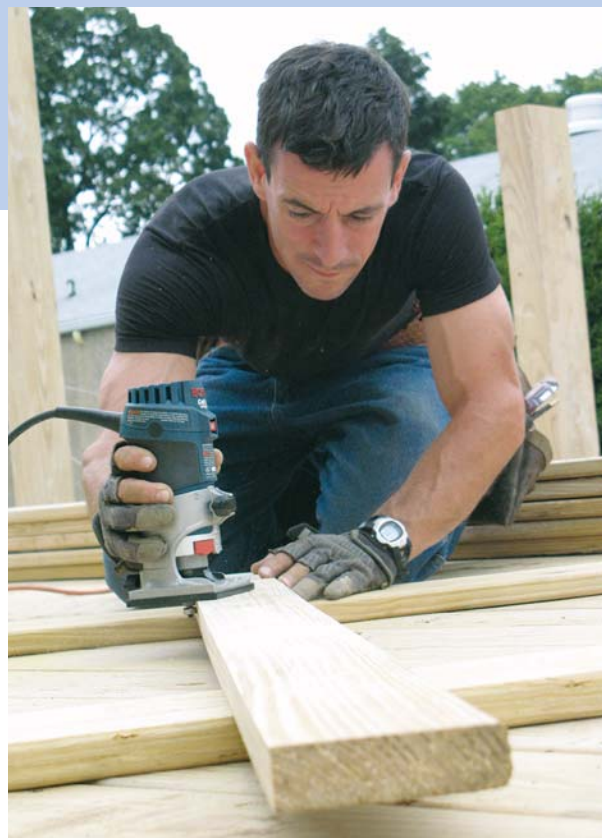
Figure 9. Often, the last (or next-to-last board, if you want the last one to be full size) must be ripped to width. Run a roundover bit in a router along the ripped edge to blend it in.
