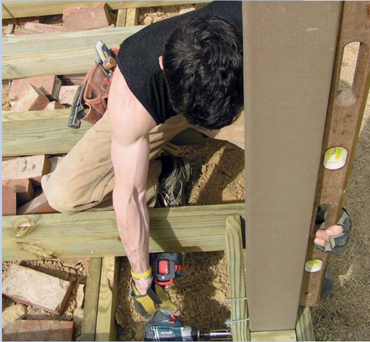
Figure 6. Use a cordless impact driver to quickly cinch down the bolts. LedgerLok screws are an alternative to bolts for wood posts, subject to local approval.
