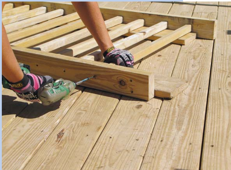
Figure 11. Spreading wood balusters out on pieces of 1-inch-thick decking centers them perfectly on 2x4 rails. An impact driver makes quick work of the 3 1 / 2 -inch screws that join the parts.
