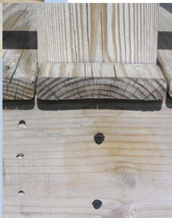
Figure 7. Using 4x6 wood posts eliminates the need to notch the ends of boards. Lay out the final location of the posts as you run the decking so that the boards and the posts are aligned. Construction adhesive and finish nails hold the outboard piece of decking in place.
