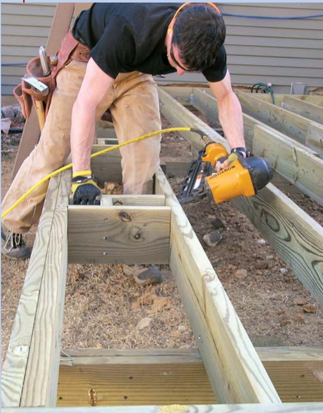
Figure 3. The post housings can be nailed or screwed into place. Locate fasteners where they won't be in the way later on when you drill for bolts.
