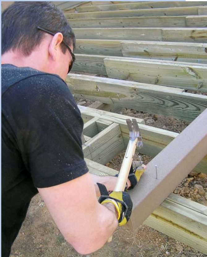
Figure 4. Nails driven partway into the post will support it at the correct height on the housing. This makes it easy for one person to plumb, shim, and bolt the post home.
