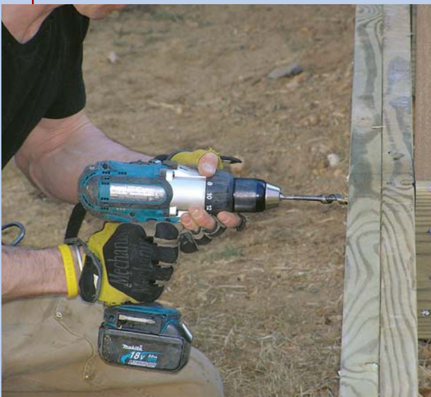
Figure 5. A heavy-duty drill and an auger bit make quick work of the bolt holes. The author drills \frac{3}{4} -inch holes for \frac{1}{2} -inch bolts to provide flexibility for shimming the post plumb.
