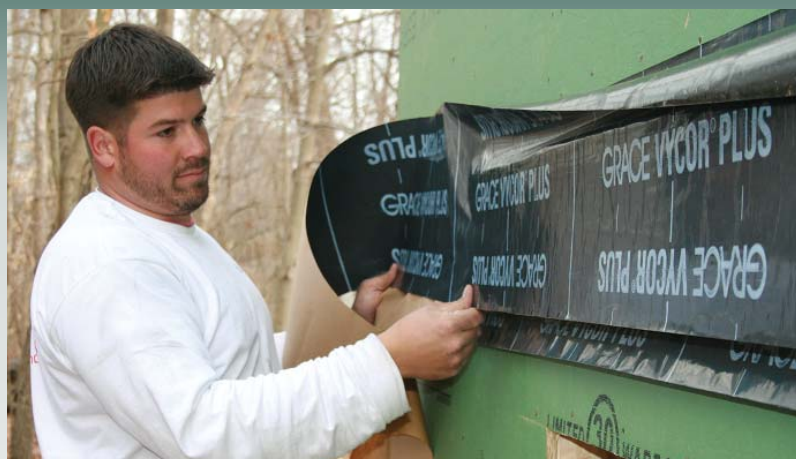
Figure 4. A second layer of peel and stick covers the installed ledger and laps up the wall. This layer protects the ledger fasteners from salt air, isolates the joist hangers from the corrosive effects of the pressure-treated ledger, and keeps water out of the joint between the top of the ledger and the wall.
