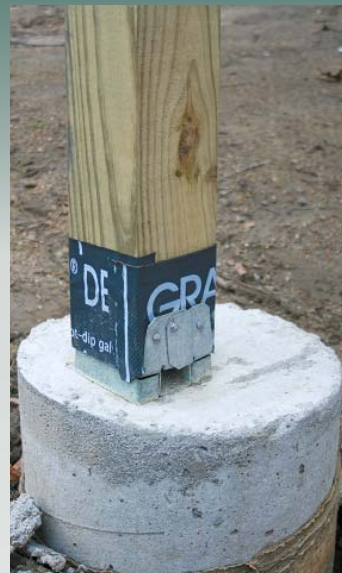
Figure 6. To isolate the framing hardware from corrosion-inducing wood preservatives, the author first wraps the wood with peel-and-stick-membrane. Finish materials will cover the membrane, both for looks and to protect it from degrading in the sunlight.
