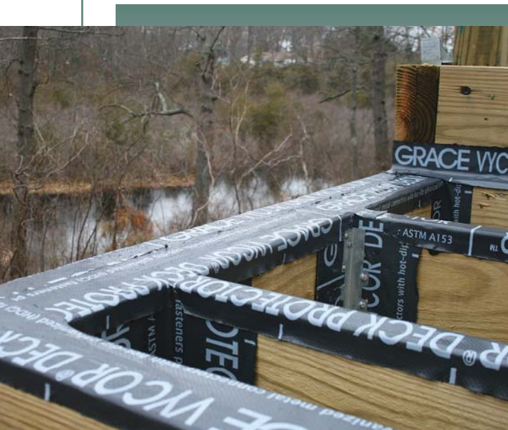
Figure 7. Even treated lumber is susceptible to rot if water is allowed to accumulate or to enter cracks. Covering the tops of joists and beams with peel and stick avoids this problem.
