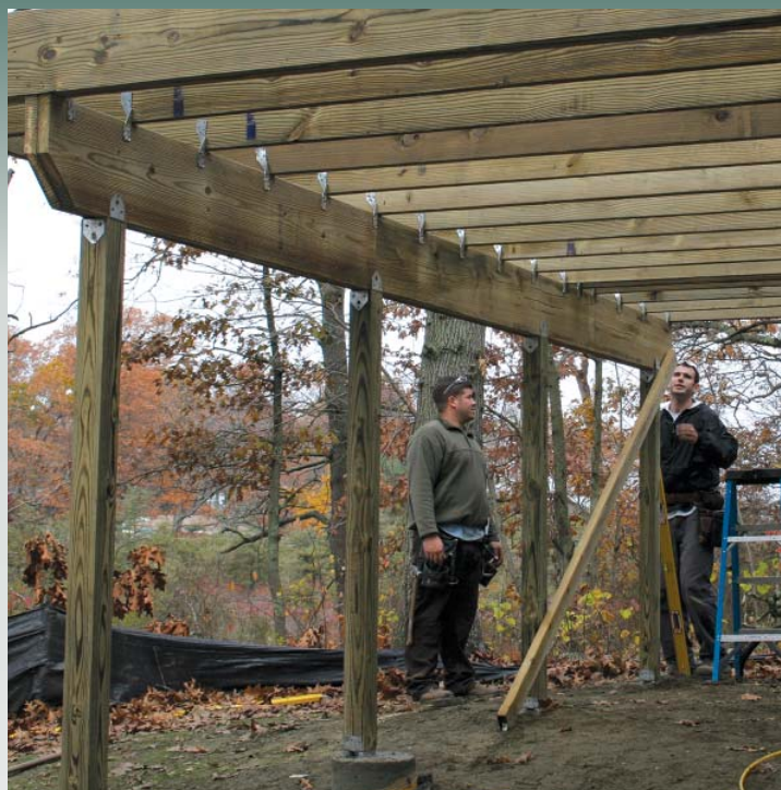
Figure 8. Because of the potential for uplift from high winds and floods in coastal areas, joists, beams, and posts must all be connected to the footings through a chain of hold-downs.
