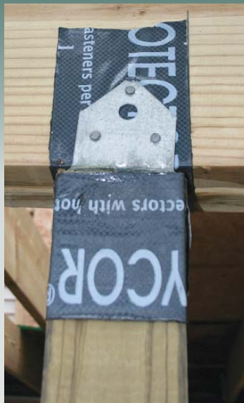
Figure 6. To isolate the framing hardware from corrosion-inducing wood preservatives, the author first wraps the wood with peel-and-stick-membrane. Finish materials will cover the membrane, both for looks and to protect it from degrading in the sunlight.
