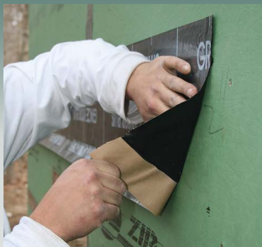
Figure 3. The first step in the ledger flashing sequence is to apply peel-and-stick membrane directly to the sheathing where the ledger will go, as shown above. The peel and stick is wide enough to extend above and below the ledger. After the siding is installed, the release film along the bottom will be removed so the peel and stick can be adhered to the face of the siding.
