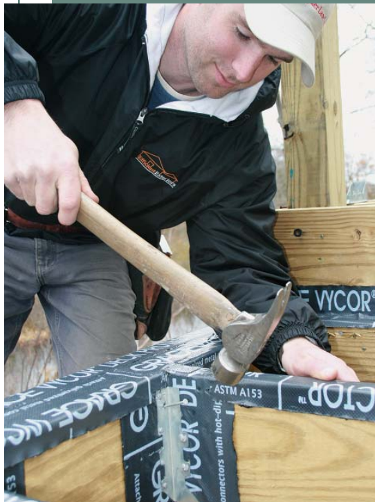
Figure 6. To isolate the framing hardware from corrosion-inducing wood preservatives, the author first wraps the wood with peel-and-stick-membrane. Finish materials will cover the membrane, both for looks and to protect it from degrading in the sunlight.
