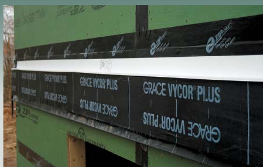
Figure 5. A corrosion-proof vinyl drip cap tops the ledger and is in turn capped by a third application of peel and stick. The sheathing used on this house has an integral weather barrier. On most houses, the building paper would lap these final waterproofing layers.
