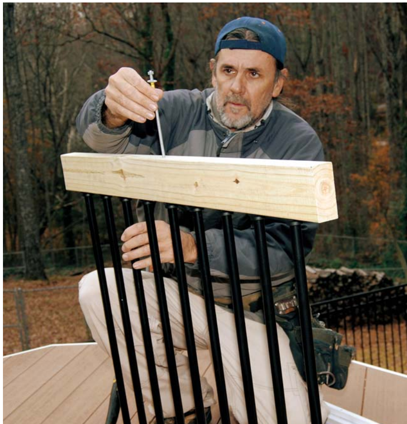
Figure 4. To firm up the assembly, the author drills a through hole at one of the central baluster connectors and runs a length of threaded rod between the upper and lower rails.
