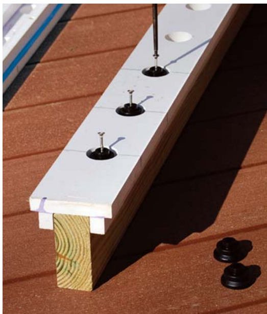
Figure 3. Lines drawn square down the side of the jig ease its alignment with the ends of the 2x4 railing. Without the lines, placing the jig to provide even spacing of the end baluster connectors would require measuring to the center of the jig's holes. To use the jig, simply place it where you want on the rail, drop in a connector, and screw.
