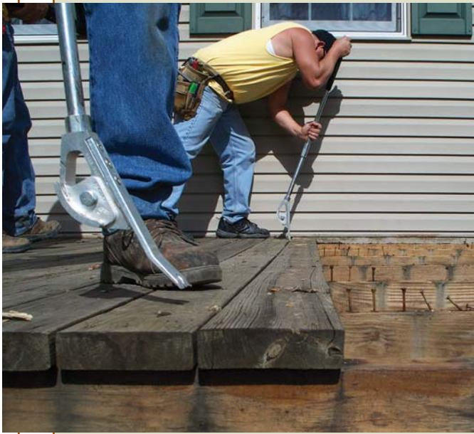
Figure 4. A variety of interchangeable heads makes the Artillery Pry Bar the author's front-line tool for demolition.
