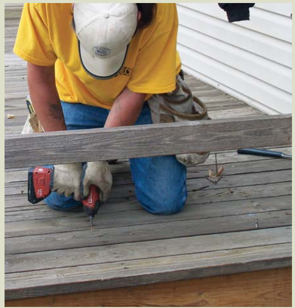
Figure 5. Screwed-down decking is harder to remove than nailed boards. Usually, 70 percent of the screws can be backed out. The rest are cut flush with the joists after the decking is pried off.
