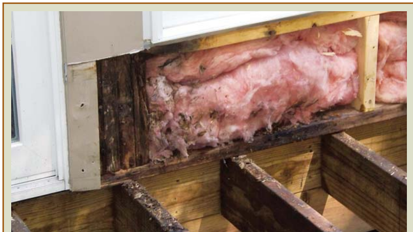
Figure 2. Most older decks aren't properly flashed to the house, but that's difficult to determine before demolition. The author includes a clause in his contract to fix such hidden conditions on a time and materials basis.
