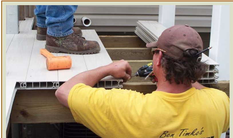
Figure 7. Low maintenance is a big selling point; the author installs only vinyl decking. Because tongue-and-groove products like the decking shown above may drain surface water slowly, it's important to ensure the framing is flat to avoid ponding.
