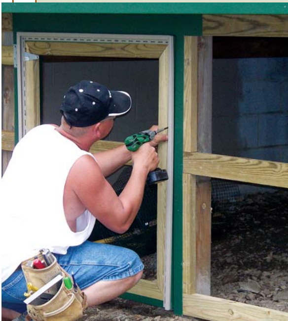
Figure 3. Enclosing or finishing the underside of the deck is a good upsell, and it makes the whole job look better by hiding the sound, but weathered, existing framing.
