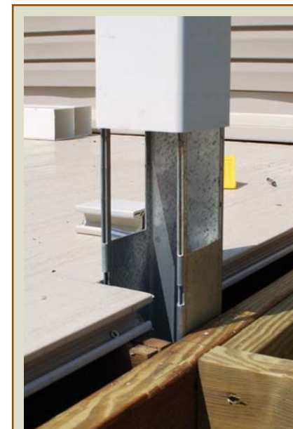
Figure 6. Post attachment is taken more seriously today than in years past. The author replaces questionable posts with a proprietary mount sold by his railing supplier.
