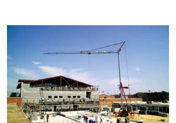
Portable Tower Crane. Working on a site too steep for wheeled machines? Check out the *Igo MA13* tower crane, which erects itself and occupies less than 12 square feet of space. It can lift nearly 4,000 pounds when the reach is 22 feet or less, and almost 900 pounds at its maximum radius (72 feet) and hook height (68 feet). You can rent one for about \$2,500 per month.
