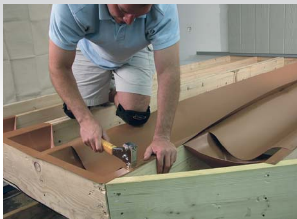
RainEscape's brown polyethylene fabric drains into a proprietary gutter system.
