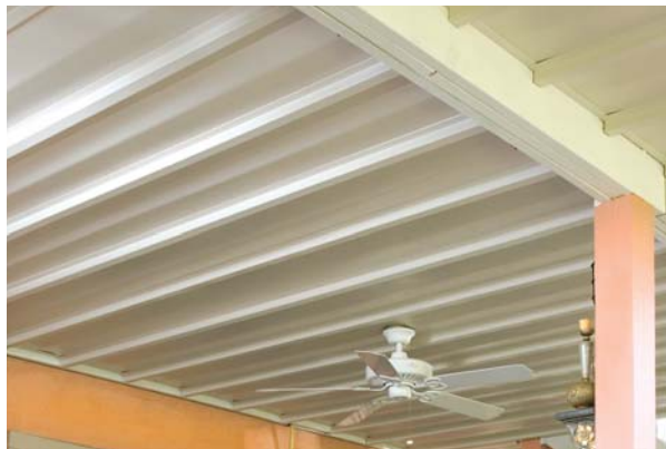
DrySpace's V-shaped vinyl panels hang from ledgers that are fastened and taped to the sides of the joists.
