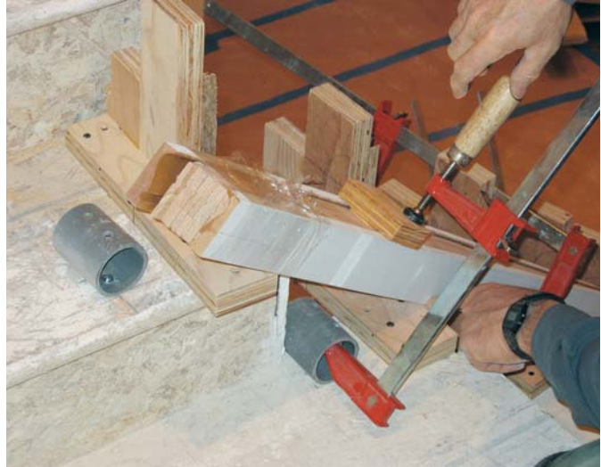
Figure 3. Short pieces of 2-inch plastic electrical conduit fastened to the floor (left) provide rugged clamping points for twisting the rail into a spiral (above).
