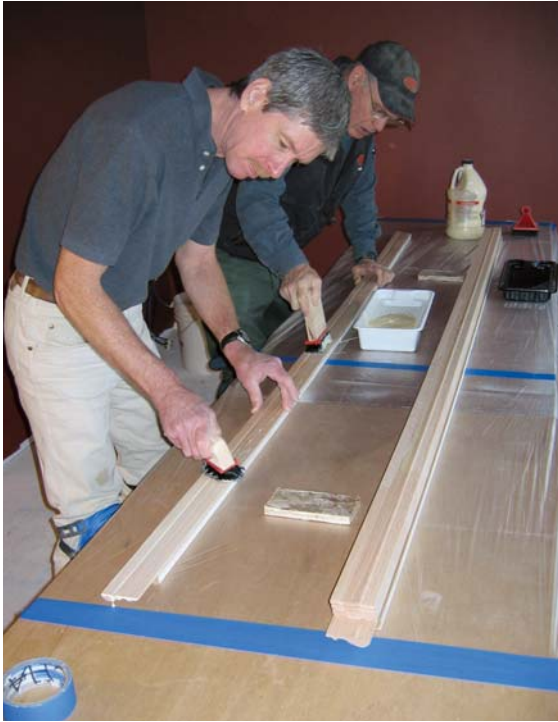
Figure 5. With the bending-rail strips stacked in order, ready to go, the author and his helper spread glue (above) and laminate the rail piece by piece (above right). With the assembly sandwiched between bending molds, they secure the bundle with plastic stretch wrap (right) to keep it from coming apart as it's being clamped to the guides on the staircase.
