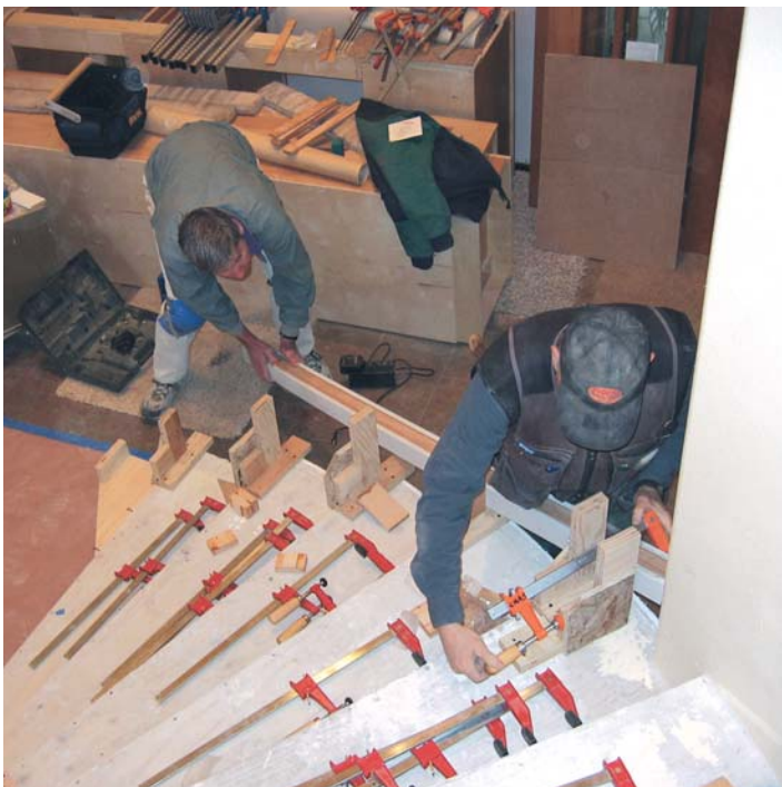
Figure 4. Before applying glue, the crew does a dry run to determine which clamps to use, where they should be placed, and whether additional clamping points will be required.
