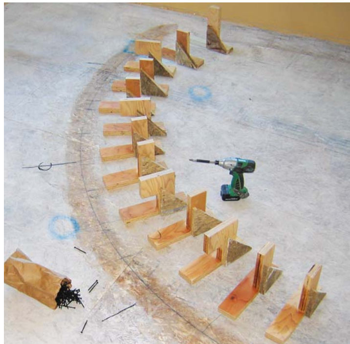
Figure 2. In preparation for making the spiral handrail, the author screws bending guides to the rough stair (above). For forming the balcony rail, he uses guides screwed to the floor of a nearby room (right).
