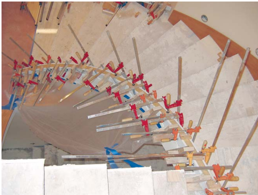
Figure 6. The rail gets clamped to the guides while the glue is wet, starting at the center and working toward the ends (top). The process takes a lot of clamps, for both squeezing the plies together and bending the assembly to the curve (left). The balcony rail is bent in a similar manner, with wood wedges providing downward pressure (above).
