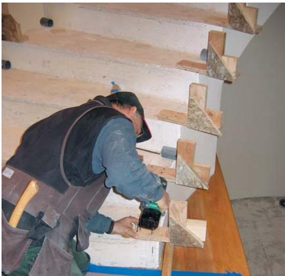
Figure 2. In preparation for making the spiral handrail, the author screws bending guides to the rough stair (above). For forming the balcony rail, he uses guides screwed to the floor of a nearby room (right).
