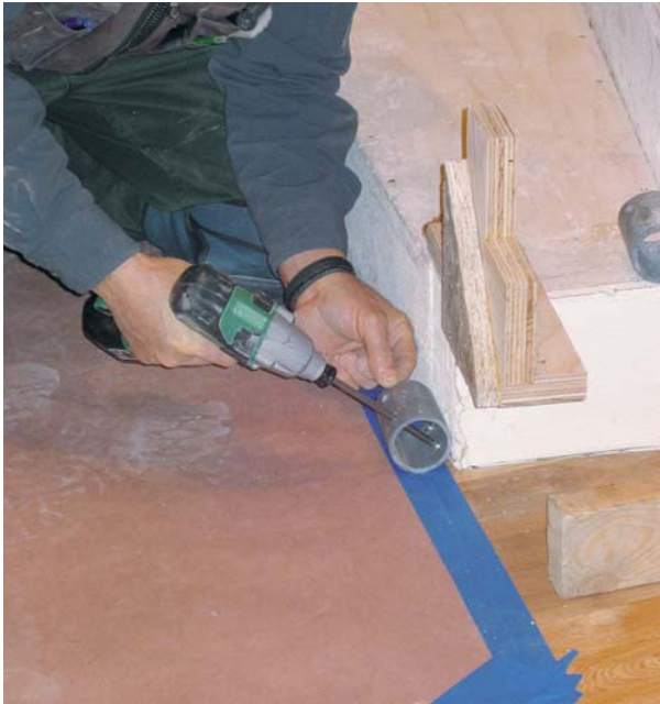
Figure 3. Short pieces of 2-inch plastic electrical conduit fastened to the floor (left) provide rugged clamping points for twisting the rail into a spiral (above).
