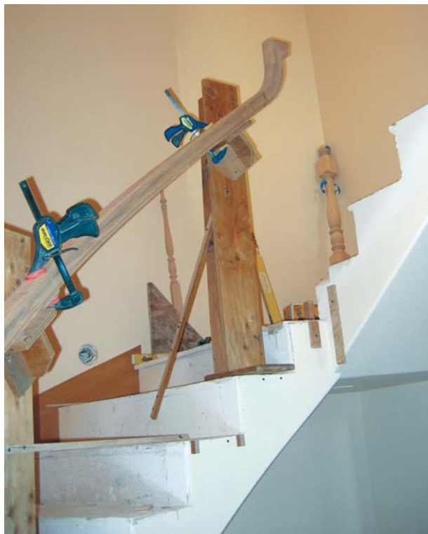
Figure 7. When the glue has cured, the author removes the clamps, scrapes and sands the rails, and then installs them with the same kinds of fittings used for straight rails.
