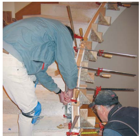
Figure 4. Before applying glue, the crew does a dry run to determine which clamps to use, where they should be placed, and whether additional clamping points will be required.
