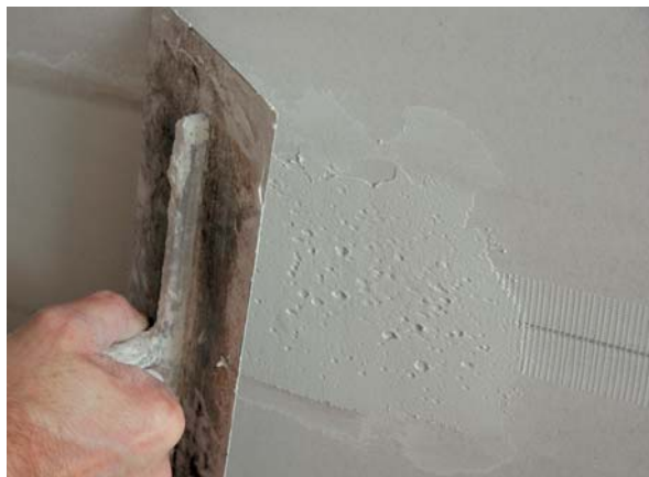
Figure 4. Since regular setting compounds can't be sanded, the author applies them in thin coats and feathers the edges (left). After the compound has set up (but before it's dry), tool marks and ridges can be shaved off with a sharp taping knife (below).
