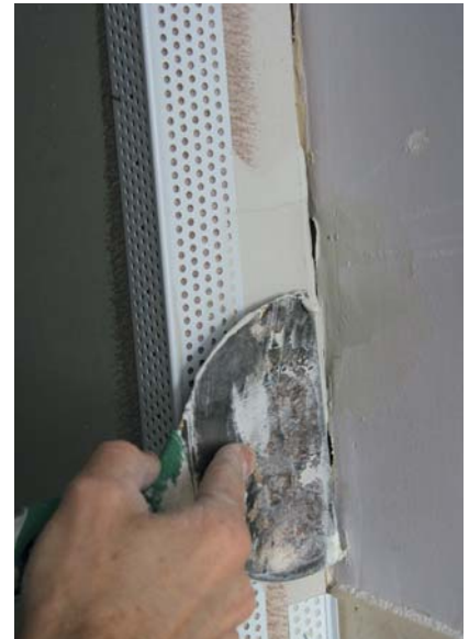
Figure 2. Setting compounds are ideal for repairing damage and filling large cracks before taping (above photos). Because of its exceptional bond strength, the author often uses setting compound when installing corner beads, which are subject to daily impacts, and when using fiberglass mesh tape, which is weaker than paper tape (left).
