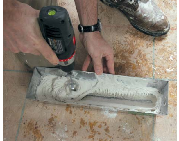
Figure 3. The author uses a mixing paddle for large batches (left) and a cake mixer mounted in a cordless drill for smaller ones (above). To avoid lumps and unpredictable results, he makes sure the water, tools, and containers are clean, and pours in the water first, then the powder.
