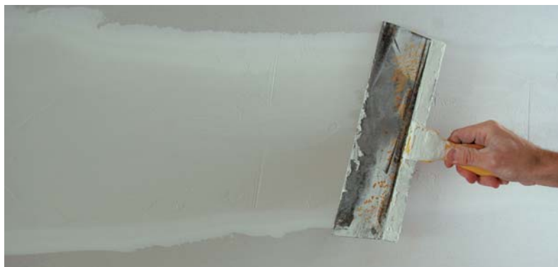
Figure 4. Since regular setting compounds can't be sanded, the author applies them in thin coats and feathers the edges (left). After the compound has set up (but before it's dry), tool marks and ridges can be shaved off with a sharp taping knife (below).
