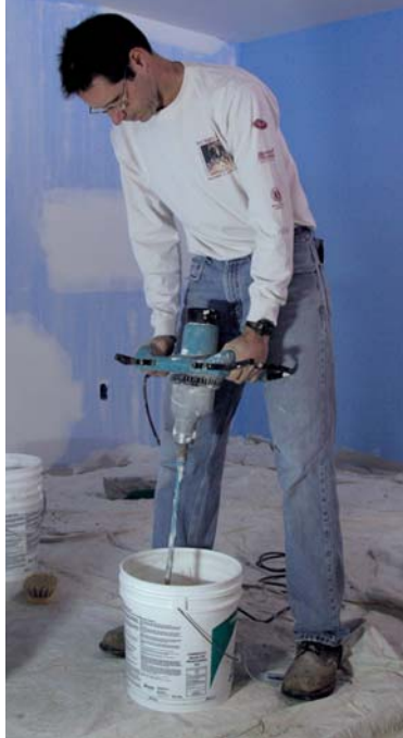
Figure 3. The author uses a mixing paddle for large batches (left) and a cake mixer mounted in a cordless drill for smaller ones (above). To avoid lumps and unpredictable results, he makes sure the water, tools, and containers are clean, and pours in the water first, then the powder.
