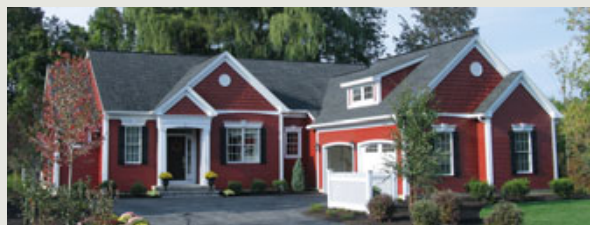
Vinyl siding qualifies for both LEED and National Green Building Standard points. This home — which is clad with Gentek vinyl siding with contoured insulation backing — was awarded LEED Gold certification in late 2008. It was built by Belmonte Builders in Saratoga Springs, N.Y.
