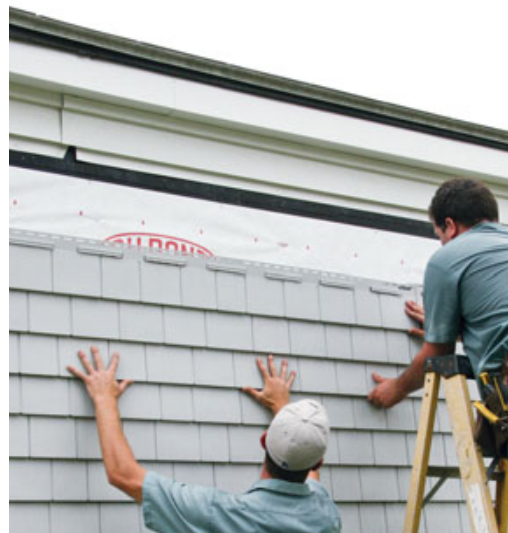
Figure 1. With injection-molded polypropylene — which takes on just about any shape — manufacturers can reproduce stone and wood siding textures more convincingly than ever before. Crane's Bellastone (above left) has real stone grit embedded in its surface. Cedar-shingle profiles are popular in the Northeast in full-coverage applications (above), while decorative shingles can be found anywhere (left).
