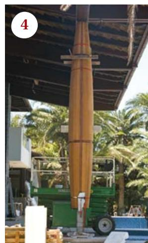
Miami's STA Architectural Group originally planned to use solid ipe for the eight columns on this high-end residence (1), which is currently under construction in Bal Harbour, Fla. But when logs of sufficient size turned out to be unattainable, the firm asked Orleans, Mass., boat-builder Suzanne Leahy to build the columns out of mahogany.
