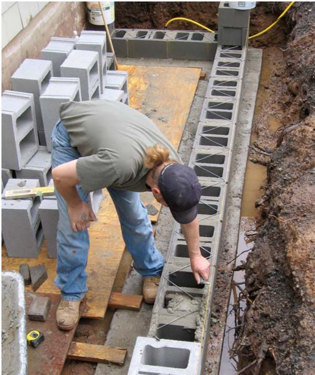
Figure 3. Blockwork starts at the corners, with the blocks laid in a full bed of mortar. Strings stretched between the corner blocks keep the courses straight. Every other course is reinforced with galvanized metal truss (above). Parging fills the pores of the block, making them more water-resistant (above right). A coat of cold asphalt supplies another layer of protection against moisture (right).
