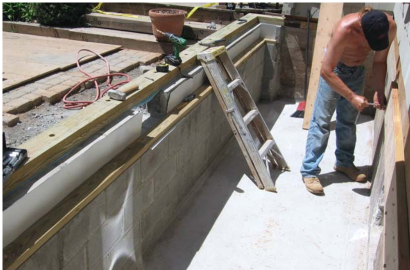
Figure 5. Switching from 12-inch to 8-inch block for the top course creates a ledge for the floor joists (above), which rest on a flashed PT sill. Full-depth blocking between the joists takes the place of a rim joist (above right). At right, the finished deck, ready for framing.
