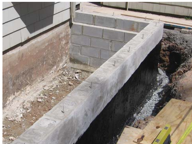
Figure 3. Blockwork starts at the corners, with the blocks laid in a full bed of mortar. Strings stretched between the corner blocks keep the courses straight. Every other course is reinforced with galvanized metal truss (above). Parging fills the pores of the block, making them more water-resistant (above right). A coat of cold asphalt supplies another layer of protection against moisture (right).
