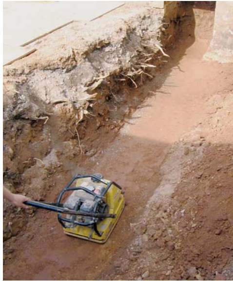
Figure 1. Before starting excavation, the author lays down sheets of plywood to protect the paver-stone patio (far left). He uses a plate compactor to prepare the soil underneath the footing (left). While he rents excavating equipment for each job, he also owns a small dump truck (below left) and an electric side-loading concrete mixer (below).
