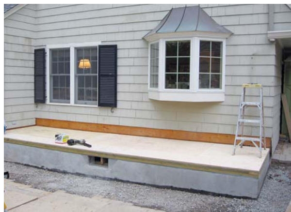
Figure 5. Switching from 12-inch to 8-inch block for the top course creates a ledge for the floor joists (above), which rest on a flashed PT sill. Full-depth blocking between the joists takes the place of a rim joist (above right). At right, the finished deck, ready for framing.
