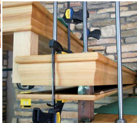
Figure 6. Temporary wooden grounds (above left) space the stone off the tread assemblies. When the stonework is done and the grounds removed, the treads will slip into the recesses with no need for scribing. The tops of the treads are screwed to the frame from below (above), then the sides and bottoms are glued in place (inset).
