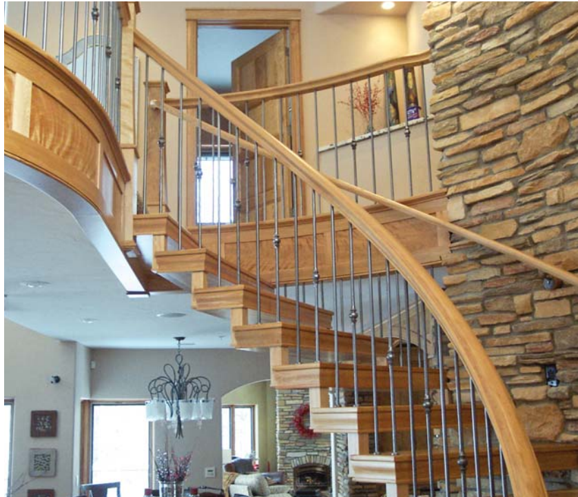
Figure 7. The lower treads of the completed stair seem to grow out of the stone (left) while the upper treads appear to hang in the air (above).
