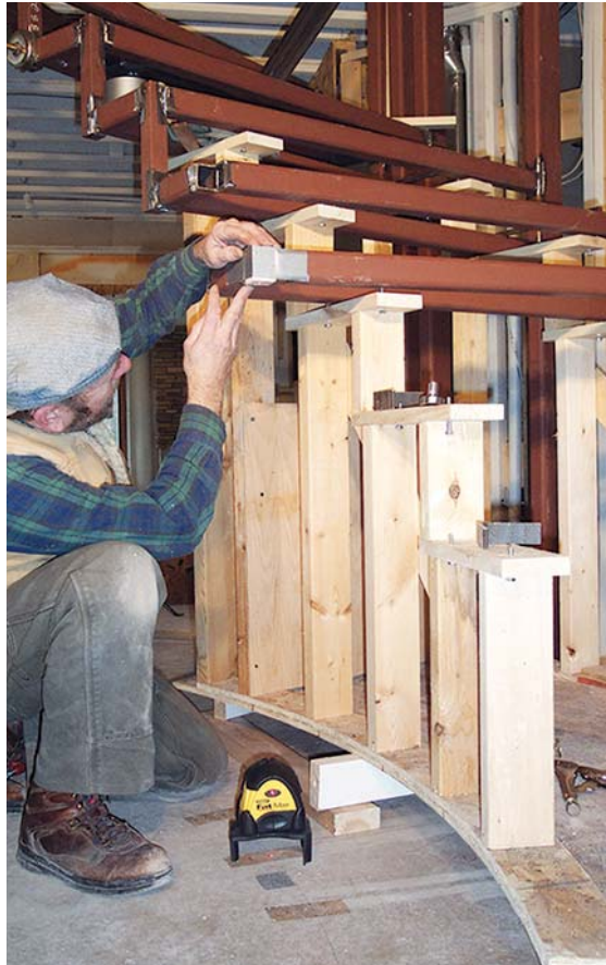
Figure 4. The author uses a temporary wooden stage to support tread frames while he positions them over the template. The block taped to the corner of this tread has the same cross section as a riser bar; its center is being used as the laser target (left). With the frame positioned horizontally in space, he checks its height against the story pole (below left). He fine-tunes the height of the frame by turning threaded bolts in the stage (below center). Once the frame is in the correct position, he connects it to the preceding tread frame by welding it to a vertical riser bar (below right).
