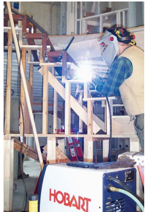
Figure 4. The author uses a temporary wooden stage to support tread frames while he positions them over the template. The block taped to the corner of this tread has the same cross section as a riser bar; its center is being used as the laser target (left). With the frame positioned horizontally in space, he checks its height against the story pole (below left). He fine-tunes the height of the frame by turning threaded bolts in the stage (below center). Once the frame is in the correct position, he connects it to the preceding tread frame by welding it to a vertical riser bar (below right).
