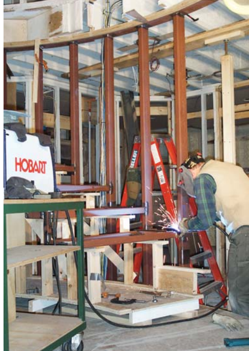
Figure 5. Posts are installed between the top and bottom plates of the wall (far left) and then welded to the tread assemblies (left). Once all the pieces are connected together, the stage is removed (below) and the welds are completed.
