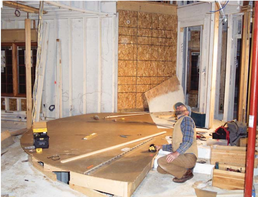
Figure 1. The author begins the new set of stairs by building a temporary platform over the basement stair opening and transferring key locations onto a hardboard template. Here he uses a laser to plumb down the location of the balcony header.
