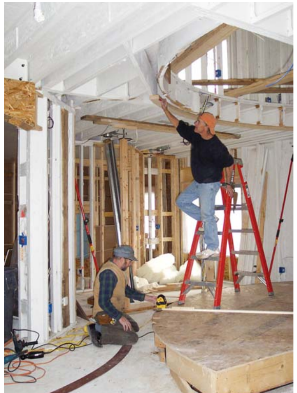
Figure 3. The curved bottom plate is located by plumbing down from a laser attached to a trammel that pivots off the center point (above). A carpenter shifts the position of the top plate so it's in line with the beam that projects up from the laser (right).
