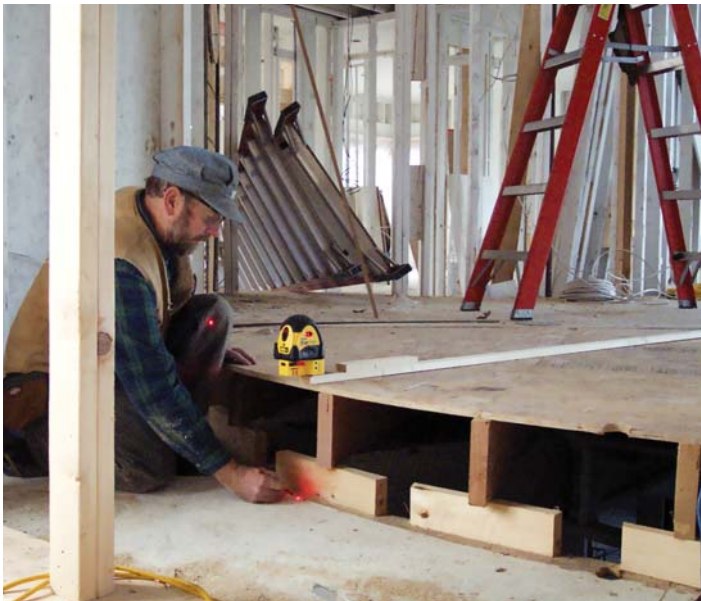
Figure 3. The curved bottom plate is located by plumbing down from a laser attached to a trammel that pivots off the center point (above). A carpenter shifts the position of the top plate so it's in line with the beam that projects up from the laser (right).
