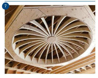
After gluing and toenailing the blocks to the framing, I added the bottom plywood sections to finish the "sandwich," trimming the edges as needed to fit into the <sup>3</sup>/4-inch step-up around the edge of the octagon. I glued and nailed the plywood in place, making sure as I went that the top and bottom circular edges were in perfect alignment (5).
