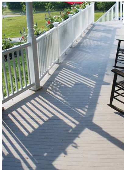
Figure 2. Correct-Porch solid T&G planks are intended for use on covered porches with sloped floors. A built-in spacer "bead" creates a small gap between planks that allows for drainage and thermal expansion. The composite can be painted or left unfinished.
