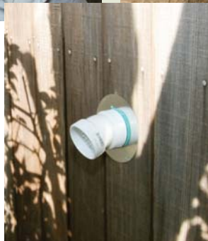
Figure 4. A plumber installs a section of flue pipe (above left), taking care to slope it so that condensate drains back to the heater. With this particular heater shown here, the flue can be ABS or PVC; in this case, it's a combination of the two (above) because the plumbers ran out of ABS. The flue passes out through the wall and terminates at a screened fitting (left).
