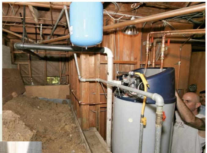
Figure 4. A plumber installs a section of flue pipe (above left), taking care to slope it so that condensate drains back to the heater. With this particular heater shown here, the flue can be ABS or PVC; in this case, it's a combination of the two (above) because the plumbers ran out of ABS. The flue passes out through the wall and terminates at a screened fitting (left).
