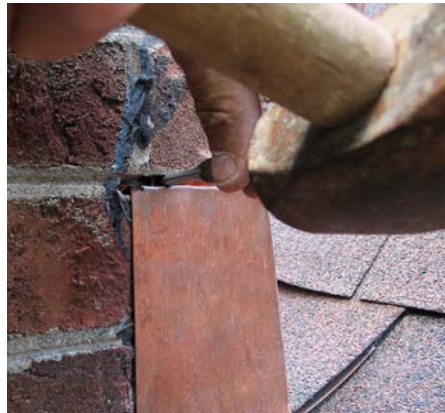
Figure 2. Counterflashings have a short “L” finished with a hook (far left). The author inserts the “L” into the kerf cut into the mortar joint, then uses a punch to tightly pack the lead strips wrapped around the hook into the kerf (left). Stainless steel sheet-metal screws fasten the counterflashings together (below).
