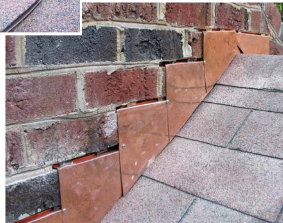
Figure 2. Counterflashings have a short “L” finished with a hook (far left). The author inserts the “L” into the kerf cut into the mortar joint, then uses a punch to tightly pack the lead strips wrapped around the hook into the kerf (left). Stainless steel sheet-metal screws fasten the counterflashings together (below).
