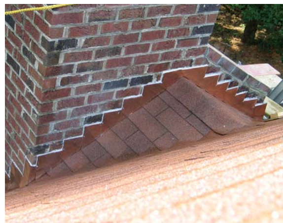
Figure 3. When caulking the vertical and horizontal edges of the counterflashing, the author uses a tuck-pointer to pack and smooth the joints and painter’s tape to keep the brick-work clean (above). The screw heads are sealed with clear silicone caulk (right).
