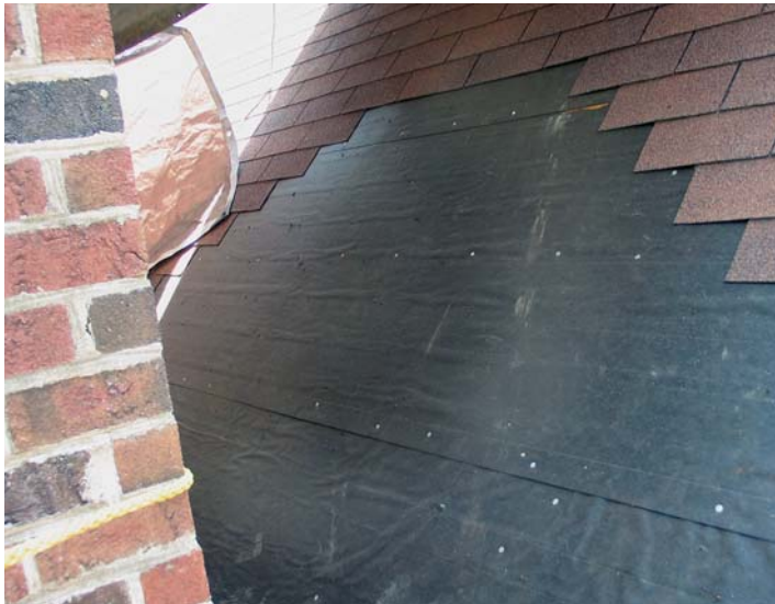
Figure 1. To make room for the cricket, the author strips the roofing around the chimney (above). A brick trowel is handy for breaking the bond between shingles without damaging them (right). The cricket is framed like a small roof; the author builds it on the ground, then installs it in one piece (bottom).
