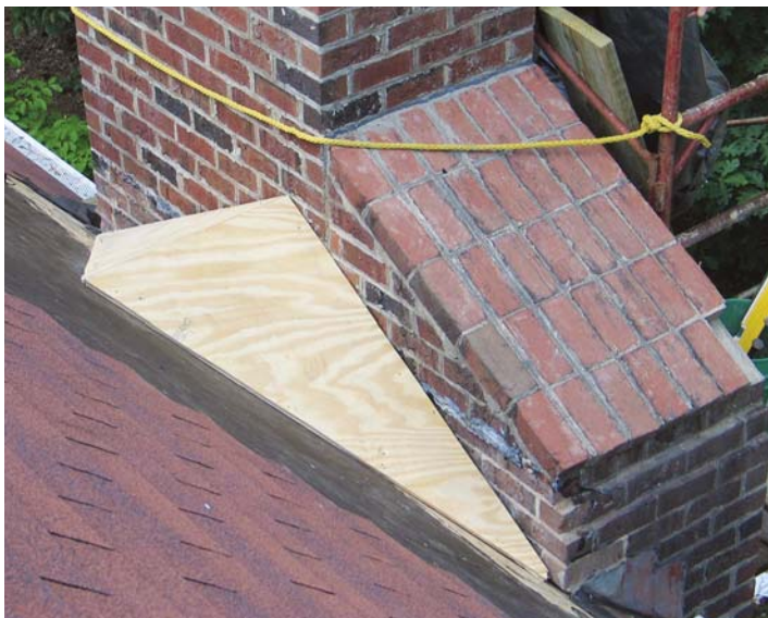
Figure 1. To make room for the cricket, the author strips the roofing around the chimney (above). A brick trowel is handy for breaking the bond between shingles without damaging them (right). The cricket is framed like a small roof; the author builds it on the ground, then installs it in one piece (bottom).
