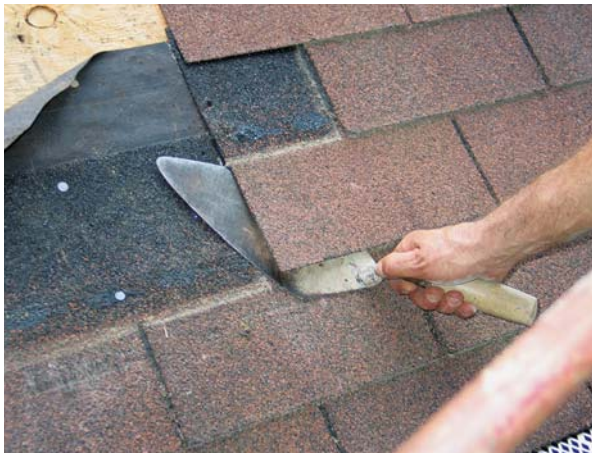
Figure 1. To make room for the cricket, the author strips the roofing around the chimney (above). A brick trowel is handy for breaking the bond between shingles without damaging them (right). The cricket is framed like a small roof; the author builds it on the ground, then installs it in one piece (bottom).
