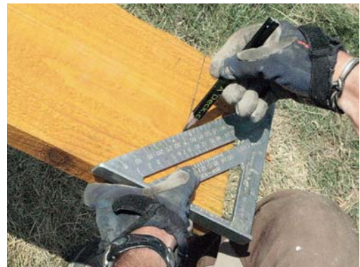
Figure 7. Rather than using a miter saw on long, unwieldy lumber, the author lays out the cuts with a square, which he then also uses to guide straight cuts with a circular saw.
