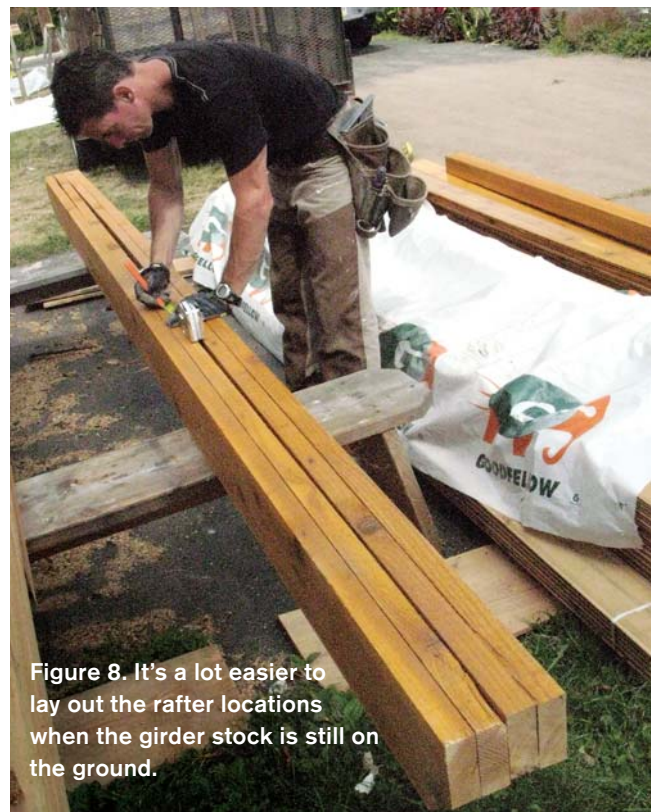
Figure 7. Rather than using a miter saw on long, unwieldy lumber, the author lays out the cuts with a square, which he then also uses to guide straight cuts with a circular saw.
