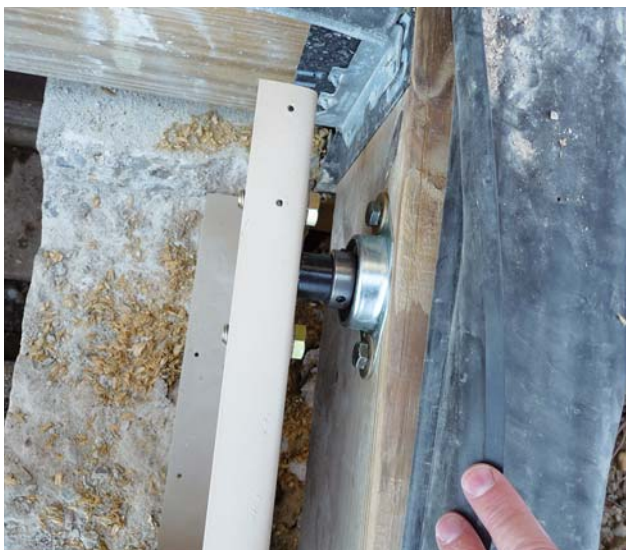
Figure 2. The 1,200-pound hatch pivots on 1-inch steel shafts supported by ball bearings.
