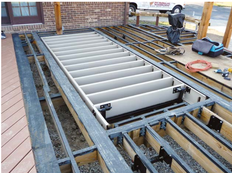
Figure 3. Steel joists make a frame that doesn't change dimension with the seasons.
