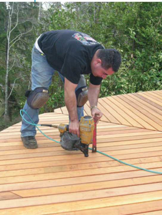
Figure 1. Nailing remains a viable and effective way to fasten decking, particularly when price is a big consideration.
