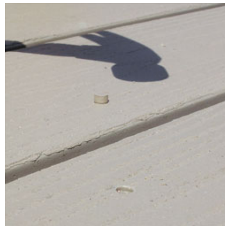
Figure 8. The Cortex system provides screws and a special driver. This combination countersinks the screw to the perfect depth for the supplied composite-decking plugs to be driven flush with the surface.
