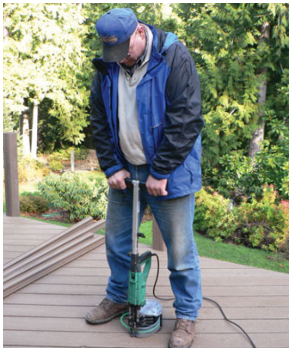
Figure 4. Nearly as fast as nailing is face-screwing with a collated-screw gun. Screws can be had with heads in a variety of colors to match most composite decking brands.
