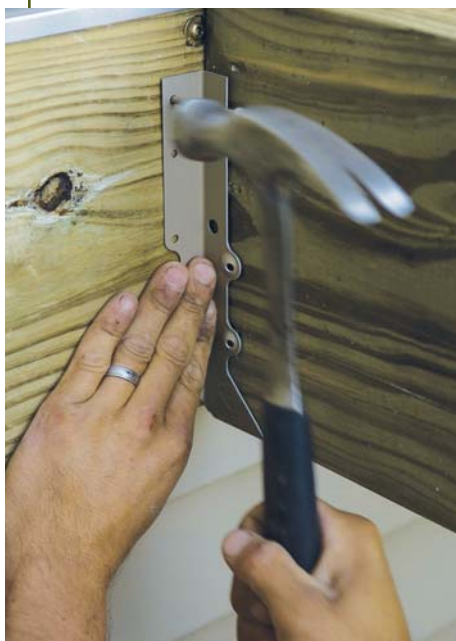
Figure 6. An alternative to hot-dip galvanization is to polymer-coat electro-galvanized steel. The polymer on this connector keeps water off the steel, preventing the galvanic reaction that causes corrosion.
