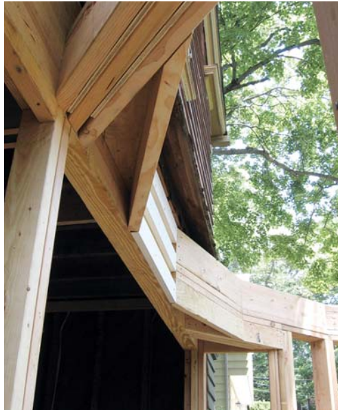
Figure 7. The interior walls at ceiling level continue the 16-sided form of the polygon, so the wall plates and box header needed to be extended to meet up with the existing wall.
