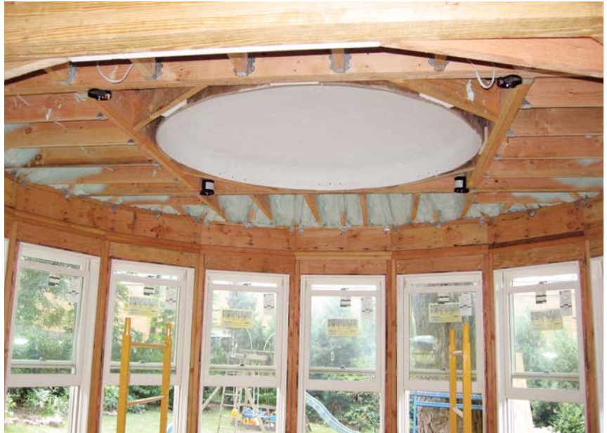
Figure 9. A beefy 2x8 grid ceiling reinforced with metal connectors helps tie the walls together while accommodating an opening for a prefabricated dome in the ceiling center. Before the dome was installed, an insulation contractor sprayed the unvented attic space with closed-cell foam insulation.
