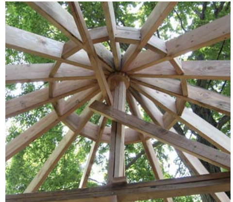
Figure 8. The 16 2x8 hip rafters were cut and installed first and bear on a 16-sided boss cut from 2x8 stock (above left). Blocking installed between the hip rafters (above) supports the other 16 common rafters, which bisect each wall section. The rafter tails, fascia, and window trim all had to match the existing frieze detail (left).
