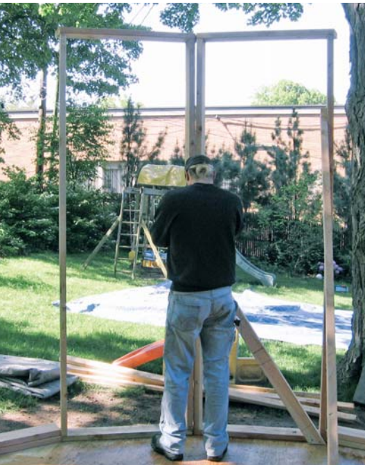
Figure 6. With rough-opening sizes that left no room for trimmers, each window wall section was a simple frame consisting of 2x6 bottom and top plates and 8-foot studs (above). A 2-by ripping fills in the triangular gap between adjacent studs at each corner (top right). An overlapping double top plate helps hold the wall sections together, while roof loads are supported by a box header installed on top of the plates (bottom right).
