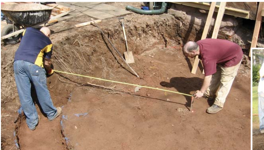
Figure 2. The addition's block foundation was built on a circular trench footing, laid out from the center point of the 16-sided polygon (above). The 12-inch-deep by 2-foot-wide footing was dug by hand in the bottom of the excavation and reinforced with rebar (right).
