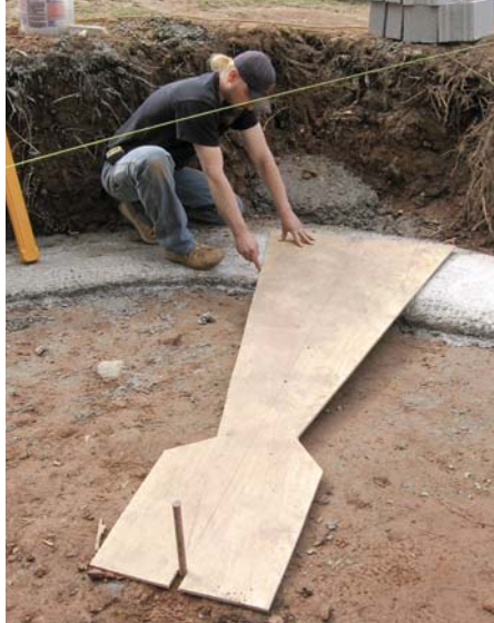
Figure 3. To lay out the foundation, the author cut a plywood template based on the dimensions of one of the isosceles triangles that make up the 16-sided polygon. The template registers against the form pin at the center of the addition; the end of the template represents each 2-foot 11^{13}/16 -inch side of the polygon.
