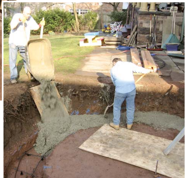
Figure 2. The addition's block foundation was built on a circular trench footing, laid out from the center point of the 16-sided polygon (above). The 12-inch-deep by 2-foot-wide footing was dug by hand in the bottom of the excavation and reinforced with rebar (right).
