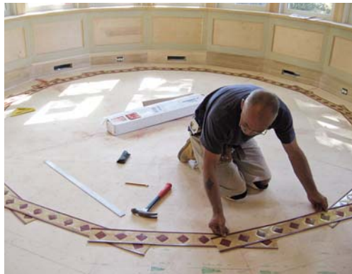
Figure 10. Each of the subtrades working on the project — from the roofer installing the soldered copper finial (top left) to the flooring contractor installing the inlaid linoleum floor (top right) — had to take into account the angles and proportions of the addition's 16-sided layout (bottom photos).
