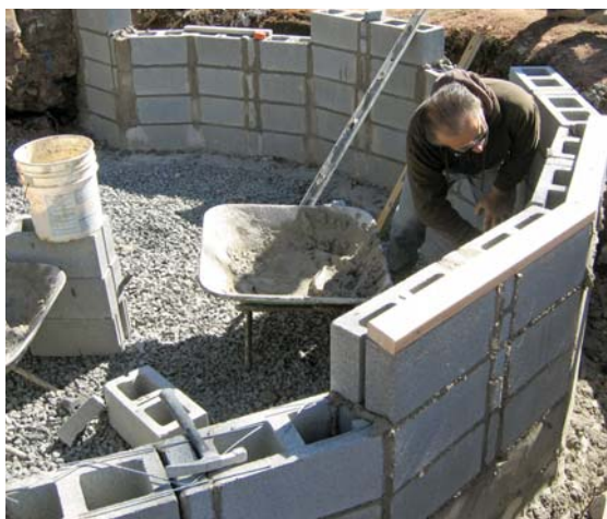
Figure 4. The stacked blockwork was reinforced with galvanized wire mesh on each course. A mock 2x4 sill cut to the exact angle and dimensions of two wall sections helped the masons get the corners right as they laid up block.
