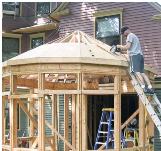
Figure 8. The 16 2x8 hip rafters were cut and installed first and bear on a 16-sided boss cut from 2x8 stock (above left). Blocking installed between the hip rafters (above) supports the other 16 common rafters, which bisect each wall section. The rafter tails, fascia, and window trim all had to match the existing frieze detail (left).
