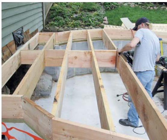
Figure 5. The rim joist was cut from 2x10 stock to match the elevation of the existing floor, but the floor joists had to be cut from 2x12 stock for the longest spans of the polygon.
