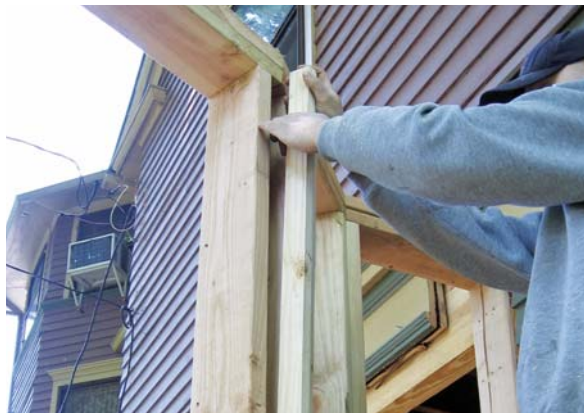
Figure 6. With rough-opening sizes that left no room for trimmers, each window wall section was a simple frame consisting of 2x6 bottom and top plates and 8-foot studs (above). A 2-by ripping fills in the triangular gap between adjacent studs at each corner (top right). An overlapping double top plate helps hold the wall sections together, while roof loads are supported by a box header installed on top of the plates (bottom right).
