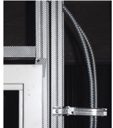
Figure 13. Nonstructural headers are made quickly by snipping channel flanges at the desired distance and folding the ends down (left). The channel tabs are then screwed to the trimmer studs (above).
