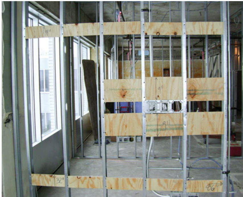
Figure 15. Wood backers provide holding power for hanging cabinets and heavy-duty shelving (above). For prehung wood doors, rough openings are formed conventionally and lined with framing lumber to supply a nailing surface (left).
