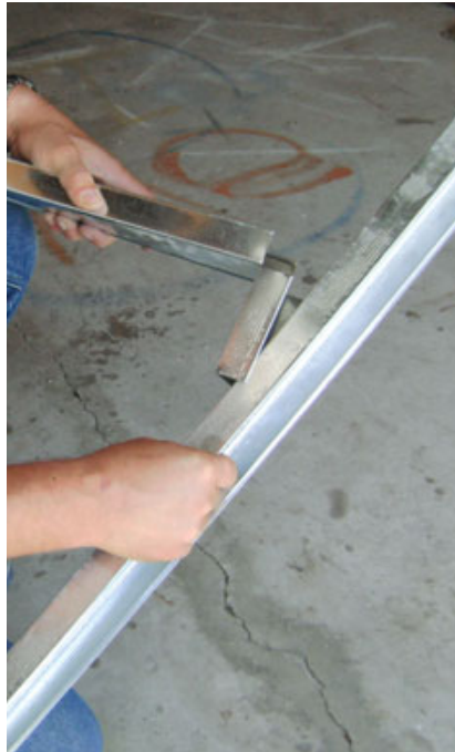
Figure 13. Nonstructural headers are made quickly by snipping channel flanges at the desired distance and folding the ends down (left). The channel tabs are then screwed to the trimmer studs (above).
