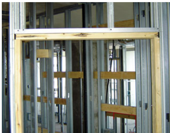
Figure 15. Wood backers provide holding power for hanging cabinets and heavy-duty shelving (above). For prehung wood doors, rough openings are formed conventionally and lined with framing lumber to supply a nailing surface (left).
