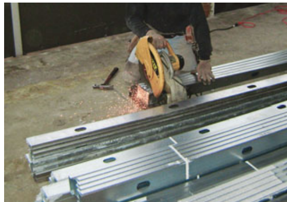
Figure 3. A 14-inch metal-cutting chop saw is handy for gang-cutting bundled studs and mandatory for cutting heavier 20-gauge steel members.
