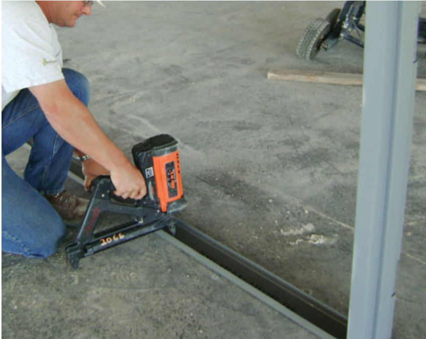
Figure 11. The bottom track is installed after all door frames are set. If shooting pins, the author uses a closer on-center schedule than when using mushroom anchors, which have better holding power in brittle concrete.
