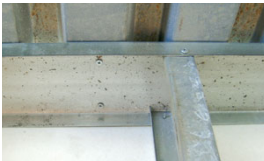
Figure 8. Self-tapping screws provide a fast, secure connection to steel roof decking. If the decking is capped with concrete, the author shoots pins instead.
