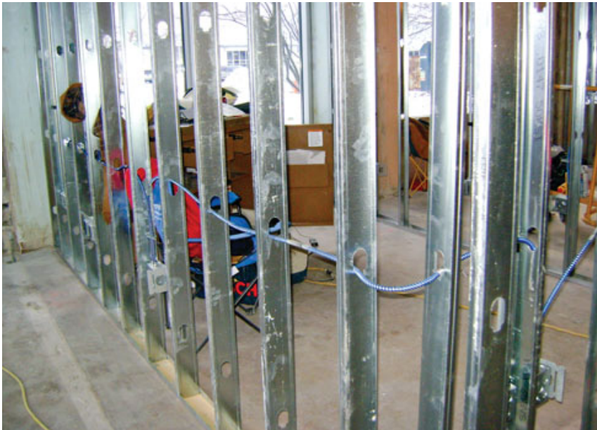
Figure 1. Getting the hang of framing with light-gauge steel studs just takes a little experience. Steel and lumber have different structural properties, but stud sizes and layout are the same (above). Deep-leg U-channel can compensate for out-of-level conditions — allowing all studs to be cut to a common length — or contain square-cut studs on raking walls (left).
