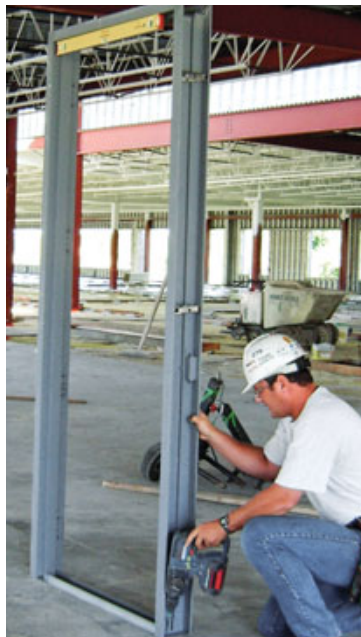
Figure 10. The author drills holes for mushroom anchors to secure a hollow metal door frame. Note the magnetic level at the head jamb (above). Plastic shims under the side jambs are used to level the head (above right). Integral tabs in the frame's side jambs provide connection points for the trimmer studs (right).
