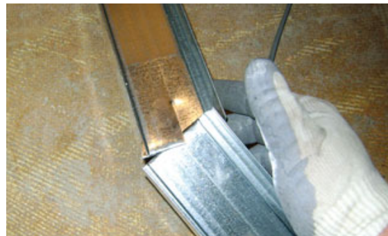
Figure 4. Inexpensive rubberized cloth gloves keep hands from getting sliced on razor-sharp cut edges. Here, a short slit in the end of one track prepares it for mating with another length.
