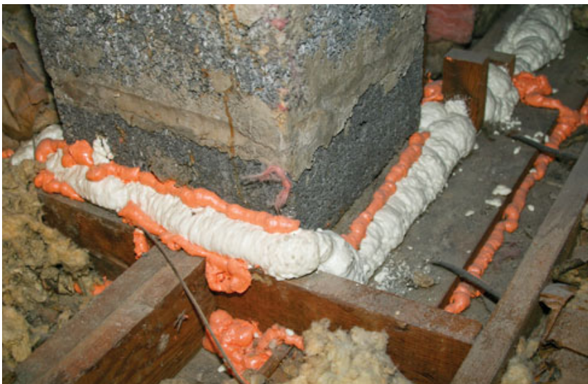
Figure 3. Can lights are covered with boxes made from duct board, which are foamed in place (top left); hvac boots are also sealed (top right). This chimney (above) was decommissioned when a direct-vent furnace was installed, so the crew has sealed around it with foam; air gaps around active chimneys are sealed using sheet metal and high-temperature silicone caulk.
