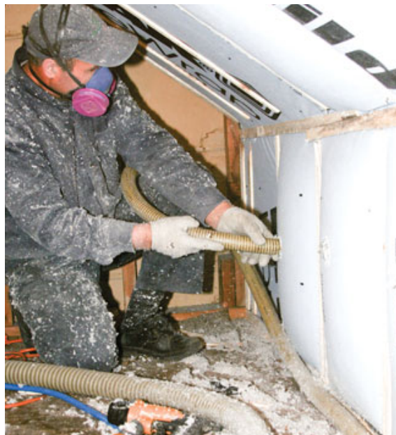
Figure 4. Here, a crew has applied housewrap to the inside face of a knee wall and low roof and is dense-blowing cellulose into the wall cavities (right) and the short sloped section of ceiling (above).
