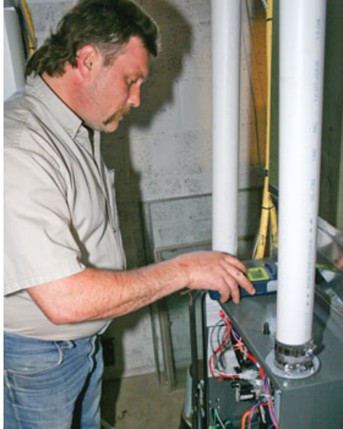
Figure 7. The technician verifies the correct operation of a new furnace and water heater (left) and documents the safety of the new kitchen range (below left). A final blower-door test (below) indicates the increase in house airtightness, from 3,600 CFM-50 to just over 1,900 CFM-50.
