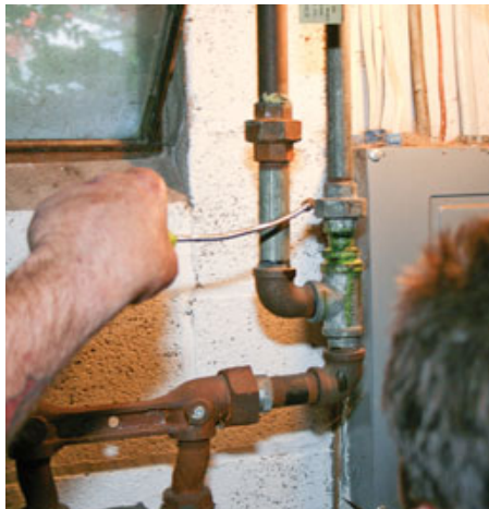
Figure 6. “Testing out” is a key element in quality assurance and customer service. In the house shown here, the technician saw the need to touch up the mastic on the basement ducts (far left). More important, he discovered a previously unnoticed gas leak (left) — a leak that probably became evident after other fittings in the piping were tightened.
