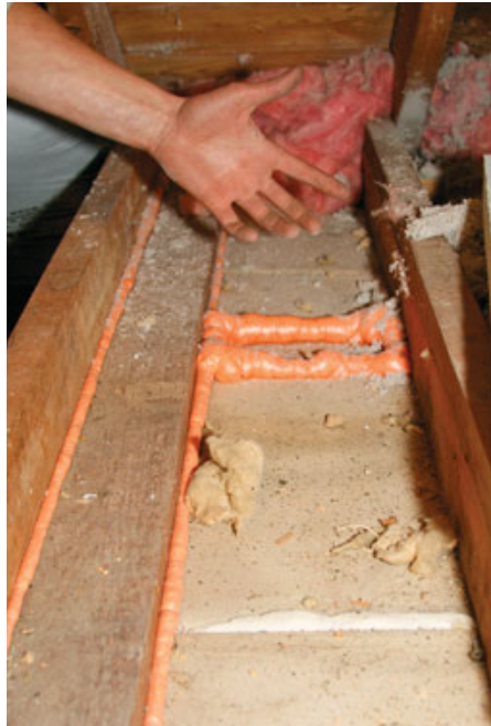
Figure 2. Crews seal spaces over cabinet soffits by installing rigid insulation across the opening at attic floor level and sealing the joints with foam (far left). Gaps where wall plates meet the attic floor must also be sealed (near left).
