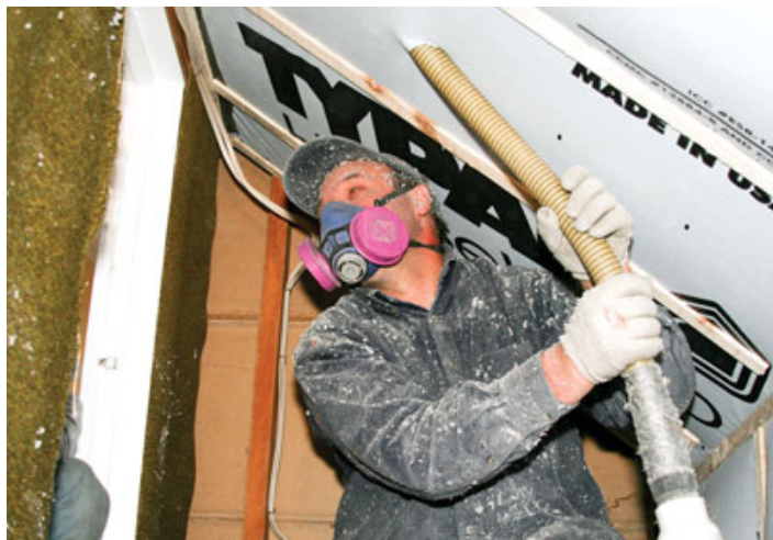
Figure 4. Here, a crew has applied housewrap to the inside face of a knee wall and low roof and is dense-blowing cellulose into the wall cavities (right) and the short sloped section of ceiling (above).
