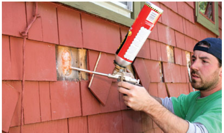
Figure 5. A GreenHomes wall-insulation crew carefully cuts off wood shingle siding to expose the sheathing (far left), then drills holes for the insulation blower hose (left). After blowing in the cellulose (below left), they seal the holes in the sheathing with closed-cell expanding foam (below), then carefully re nail the shingles.
