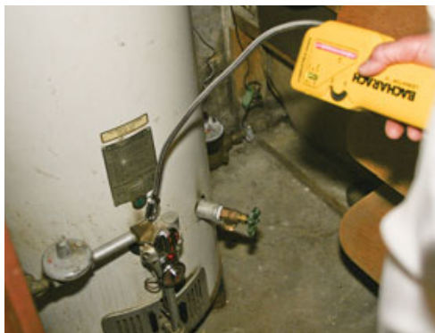
Figure 1. After drilling holes to insert sensor probes in the appliance flues (top left), the advisor uses a combustion analyzer to check for complete combustion in the furnace and water heater (top right). With doors and windows shut and all exhaust fans in the building operating, he uses a manometer to check the draft (bottom left); he is also required to check gas piping for leaks (bottom right).
