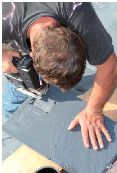
Figure 2. Authentic Roof slates can be scored with a utility knife and snapped (above), or cut with a jig-saw (right). A Shingle Shark makes quick work of repetitive cuts (far right).
