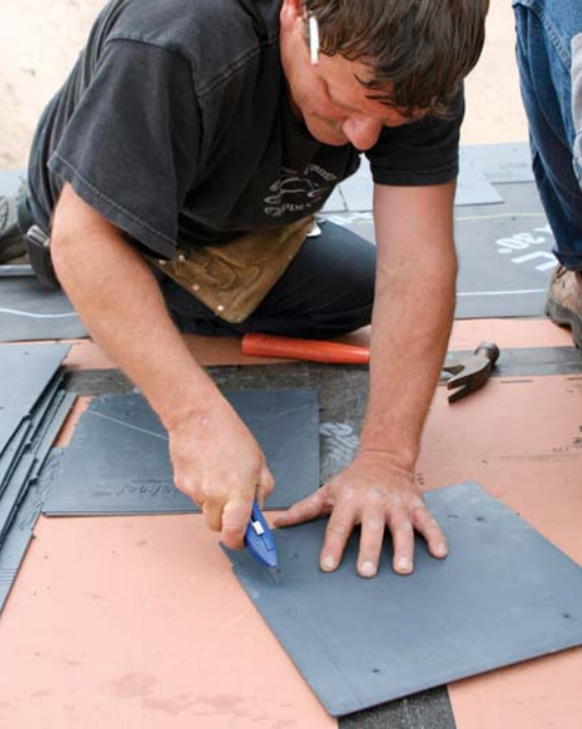
Figure 2. Authentic Roof slates can be scored with a utility knife and snapped (above), or cut with a jig-saw (right). A Shingle Shark makes quick work of repetitive cuts (far right).
