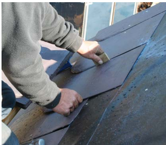
Figure 6. Like natural slate, synthetic slates have slight color variations, so bundles must be mixed before installation (above). To keep the decorative rounded slates in alignment with the field slates, the author uses a spacer block (left).
