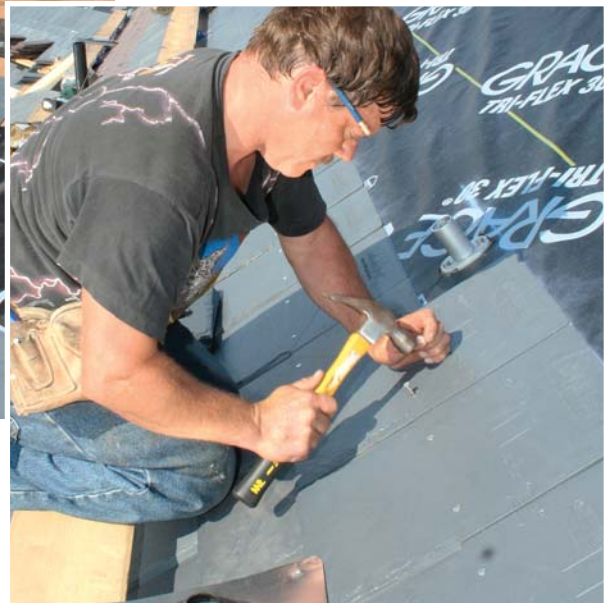
Figure 5. Valleys are lined with peel-and-stick underlayment before the 26-gauge galvanized metal W-flashing is installed; the slates butt directly against the rib in the flashing (above). Since they can't be installed with a pneumatic nailer, the slates are hand-nailed (right).
