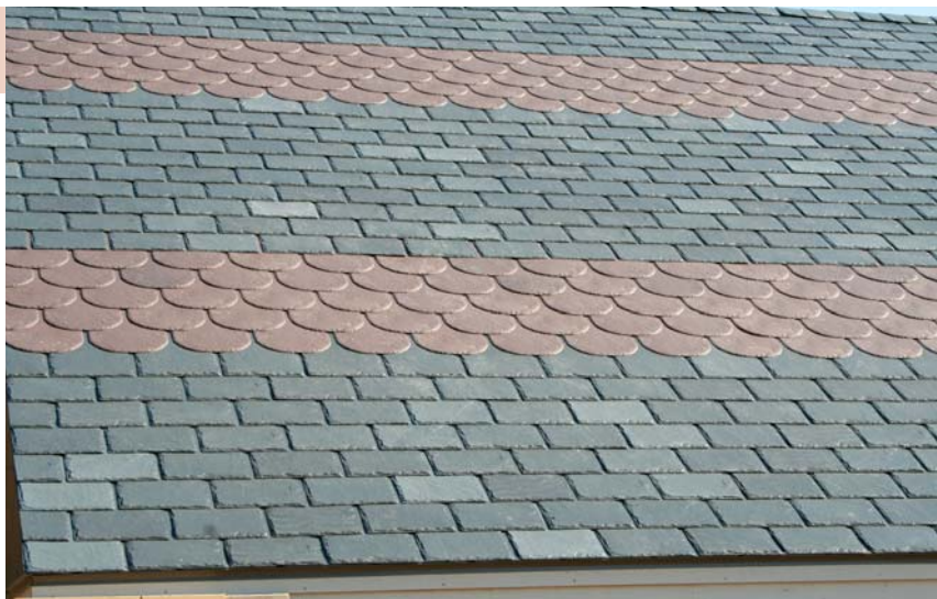
Figure 6. Like natural slate, synthetic slates have slight color variations, so bundles must be mixed before installation (above). To keep the decorative rounded slates in alignment with the field slates, the author uses a spacer block (left).
