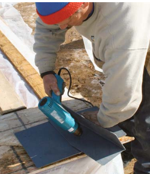
Figure 8. In cold weather, the slates are stored in a warm area and heated to above 50°F so they're easier to cut (top). Cap slates — which have a ridge channel molded into the back — are warmed with a heat gun, then bent into shape (above) and nailed into place at a hip or the ridge (right).
