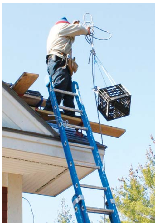
Figure 3. The slates weigh about the same per square as asphalt shingles, but they're much bulkier. Here, the author uses a milk crate to stock the roof a dozen pieces at a time.
