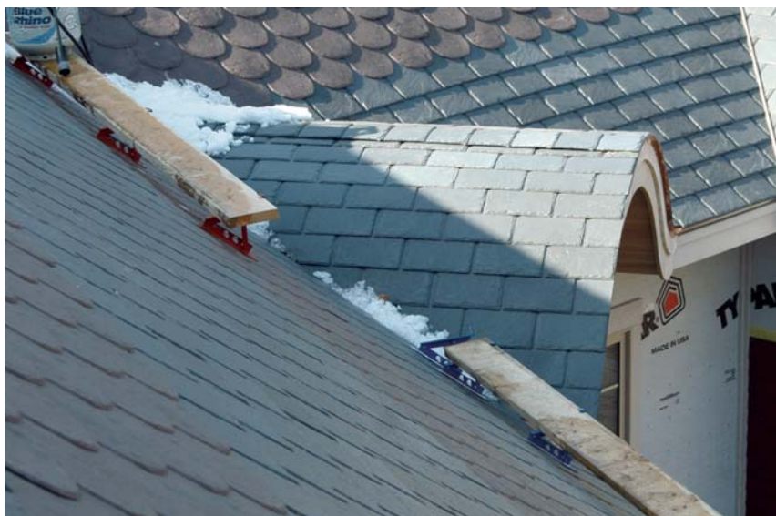
Figure 7. Authentic Roof slates can be heated up and molded to fit such curved shapes as barrel-vaulted roofs.
