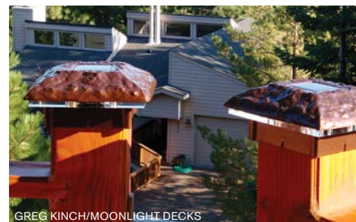
Figure 2. The easiest lighting to install is solar powered. Although the caps can look great, the light from the LED bulbs may seem cold.
