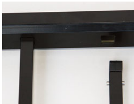
Figure 8. The Durarail system is made from heavy powder-coated aluminum; here it's shown with a combination of pickets and tempered glass (above). The balusters in CertainTeed's Durham system (right) are held in the rails by spring-loaded pins; the compressible rubber end piece prevents rattling.
