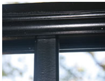
Figure 2. Co-extruded material has a wood-vinyl composite capped by a thin layer of vinyl (top). The mottled appearance of the single-layer composite at far left (in above-left photo) is due to the presence of partially exposed wood fiber; the cap layer of the co-extruded material to its right contains no fiber. The cap layer on the GAF RailWays product (above-right photo) has the texture of wood that's been painted and back-rolled.
