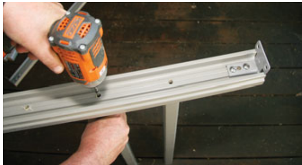
Figure 3. Like many composite products, the Azek Premier Rail system is installed by sliding a post sleeve over a wood support post (far left), screwing balusters to a subrail (left), covering the subrail with a top rail (below left), and then securing the rails to posts (below).
