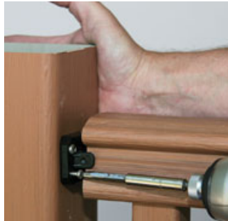
Figure 7. With the lower rail of the Veka VI Pro system in place and the balusters in their holes (far left), all that's left to do is fit the upper ends of the balusters into the top rail. The VI Pro uses heavy aluminum hardware (above left); plastic hardware — as on the CertainTeed Panorama rail (left) — is more typical for vinyl railings.
