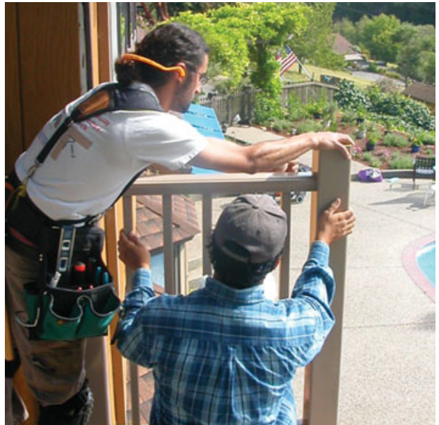
Figure 3. Like many composite products, the Azek Premier Rail system is installed by sliding a post sleeve over a wood support post (far left), screwing balusters to a subrail (left), covering the subrail with a top rail (below left), and then securing the rails to posts (below).
