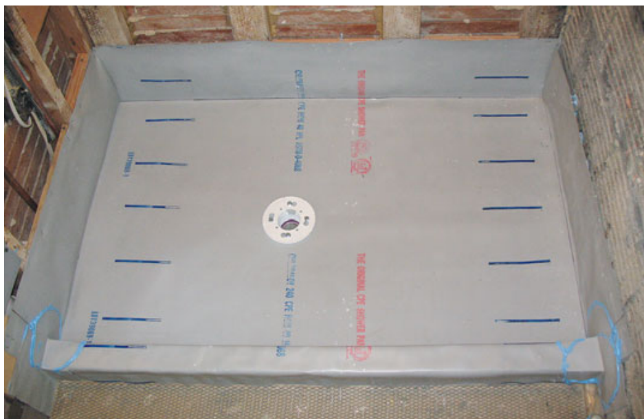
Figure 8. The liner must be slit where it runs over the curb (above left). Rectangular patches of Chloraloy bedded in Noblesealant help to waterproof the jambs (above center), but there is still a tiny hole at the inside corner where the jamb meets the curb. A preformed outside-corner dam from the manufacturer seals this spot (above right). Having passed a water test, the completed liner is ready for installation of the wall substrate and setting bed (left).
