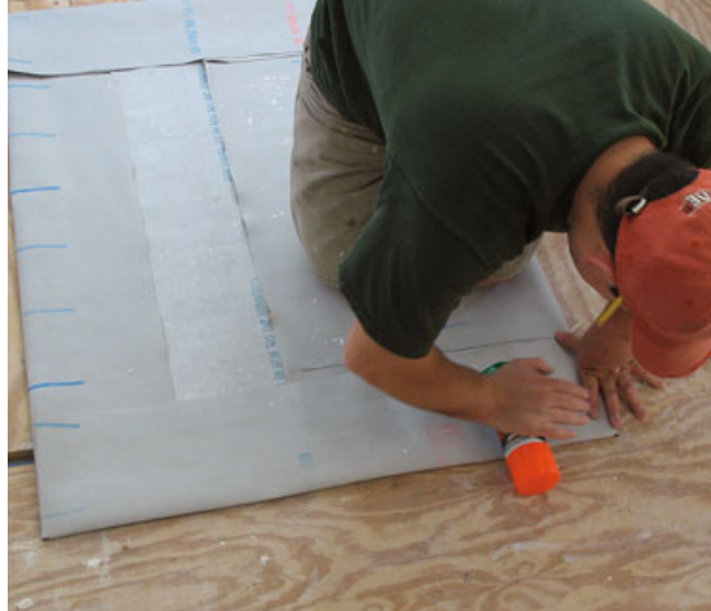
Figure 5. With the shape of the shower floor and sides of the pan marked on the Chloraloy, the liner is cut to size (left) and creased along the lines where the walls and curb meet the floor (above).
