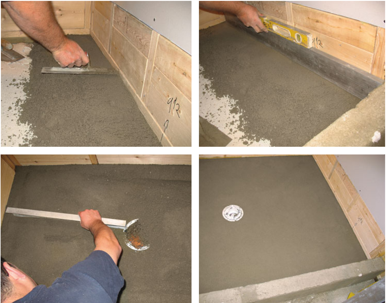
Figure 4. After skimming the concrete slab with a bond coat of thinset, the tile setter packs a mortar screed along one of the walls (top left), then checks to make sure that it's straight and level (top right). Next, he makes screeds all the way around the shower, then fills toward the center, taking care to create a straight slope between the screed and the drain (above left). When complete, the mud bed is level at the perimeter and slopes at least \frac{1}{4} inch per foot toward the drain (above right).
