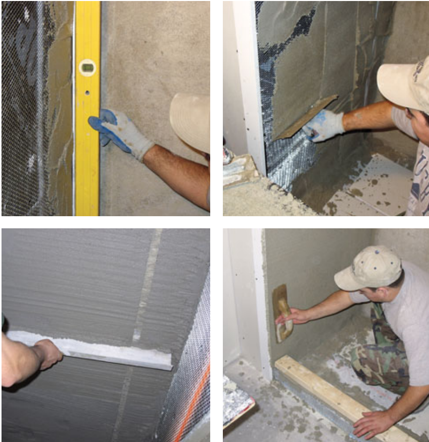
Figure 10. An aluminum float strip is pressed into the mortar along each side of the wall, then straightened and plumbed with a level (top left). After the remaining area has been built out with mortar (top right), the wall is screeded flat by pulling and sawing an aluminum angle along the face of the float strips (above left). The float strips are removed, the recesses are filled in, and the surface is smoothed with a float or trowel (above right).
