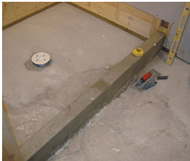
Figure 2. On wood-framed floors, the author makes the rough curb from 2x4s (left); on a slab, he lays brick, then skims it with thinset (right).
