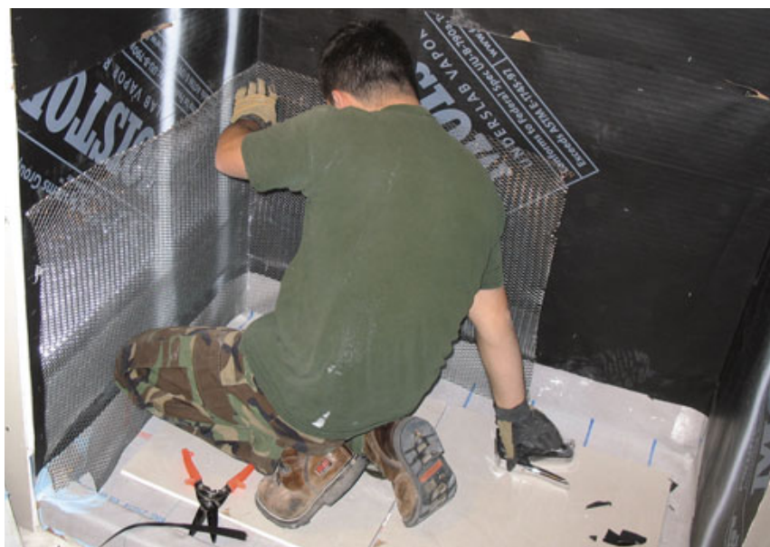
Figure 9. In preparation for mortar, the wall is covered with a moisture-resistant membrane, followed by a layer of expanded metal lath.
