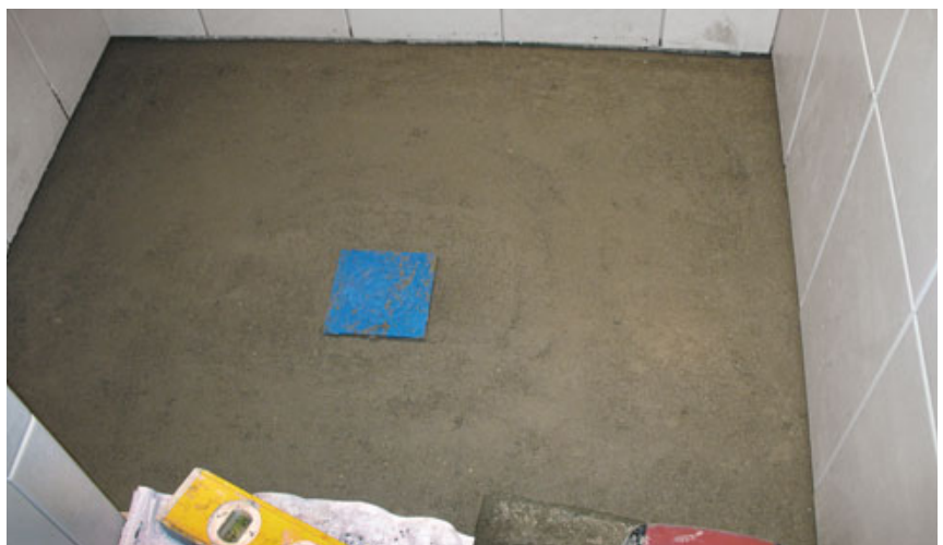
Figure 12. The setting bed is installed in much the same way as the mortar under the liner: Screeds are built up around the perimeter (top) and material is packed in toward the drain (center). The top surface of the completed setting bed (bottom) should be slightly more than one tile thickness lower than the wall tile and drain.
