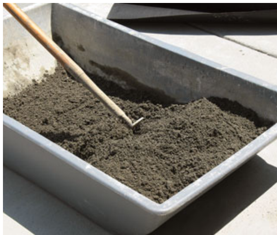
Figure 3. Deck mud is mixed dry and crumbly so that it holds its shape. It can then easily be packed and scraped to the desired slope.
