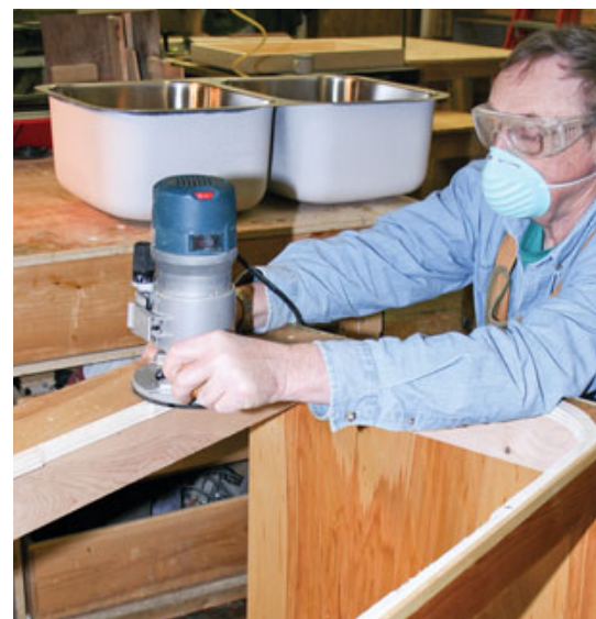
Figure 6. Instead of hanging undermount sinks from a stone countertop, the author rabbets the sink opening in the plywood top of the cabinet before the cabinet is installed.
