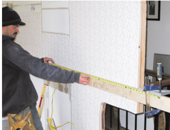
Figure 1. Horizontal layout sticks provide an accurate record of room dimensions and details; later, they'll also be used to lay out the kickspaces during cabinet installation (left, top). Cut to the height of a cabinet, the drawer layout stick gives key construction details, including the top and bottom of the carcass, the size of each drawer, the position of the slides, and the size of the applied drawer fronts (bottom).
