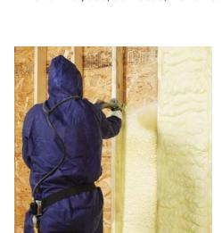
**Spray-On.** Icynene's water-blown *LD-R-50 Spray Foam Insulation* expands to 100 times its applied thickness to completely fill wall and rafter cavities. It does double-duty as a built-in air barrier, and the open-cell foam is water-vapor-permeable. This new formula uses a castor-bean oil ingredient to reduce its petroleum-based content and has an R-value of 3.7 per inch. Installation by a licensed dealer costs 65 cents per inch thickness per square foot.
