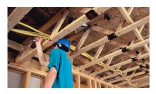
**Trimmable Truss.** Universal Forest Products says its *Open Joist* has a higher strength-to-cost ratio than any other engineered floor joist and can even beat the cost of lumber joists in some designs. Plus, the open web truss construction gives mechanical subs better access, says the company. Joists come in four depths; lengths up to 30 feet can be ordered in 1-foot increments and trimmed up to 5½ inches per side. The 11½-inch depth costs \$1.50 per linear foot.
