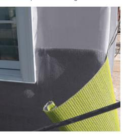
provide drainage and ventilation. The fabric remains breathable even when covered with mortar or a scratch coat. Formerly called Mortairvent, it is sold in 200-square-foot rolls for about \$150.
