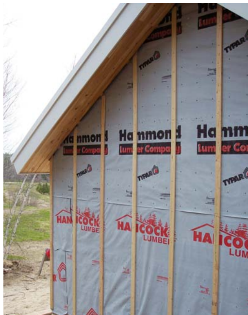
Taggart installs rain screens to keep water out of walls and prolong the life of trim, siding, and paint.
