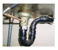
The drain connection at the wall is too high on this sink, resulting in a 9-inch-deep trap seal — 5 inches deeper than is allowed by code.
