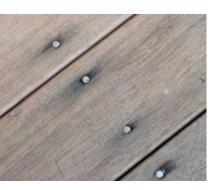
The mahogany decking we installed on a house last year has developed some dark staining around the stainless steel nail heads (see photo). The staining is worse on the front porch, which is covered, and not nearly as bad on the back deck, which receives full sun. What's causing it?
